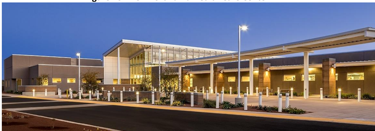
Figure 13: New Fort Yuma Health Care Center
