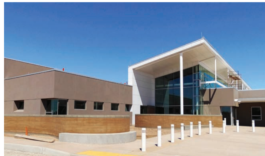
Figure 3-10. Fort Yuma under construction with rammed earth walls
