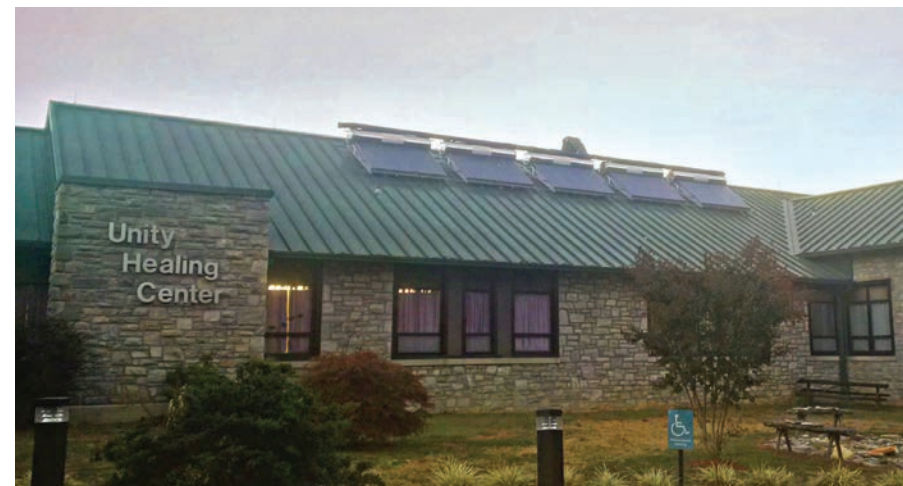
Figure 4-3. The Unity Healing Center with rooftop PV panels
