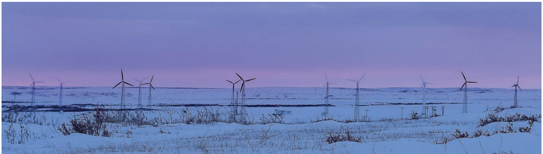
Figure 3-6. The Kotzebue Electric Association Wind Farm
