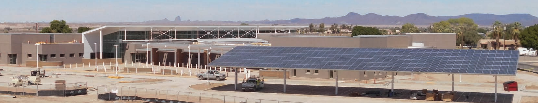
Figure 3-9. Fort Yuma under construction with PV panel shaded parking
