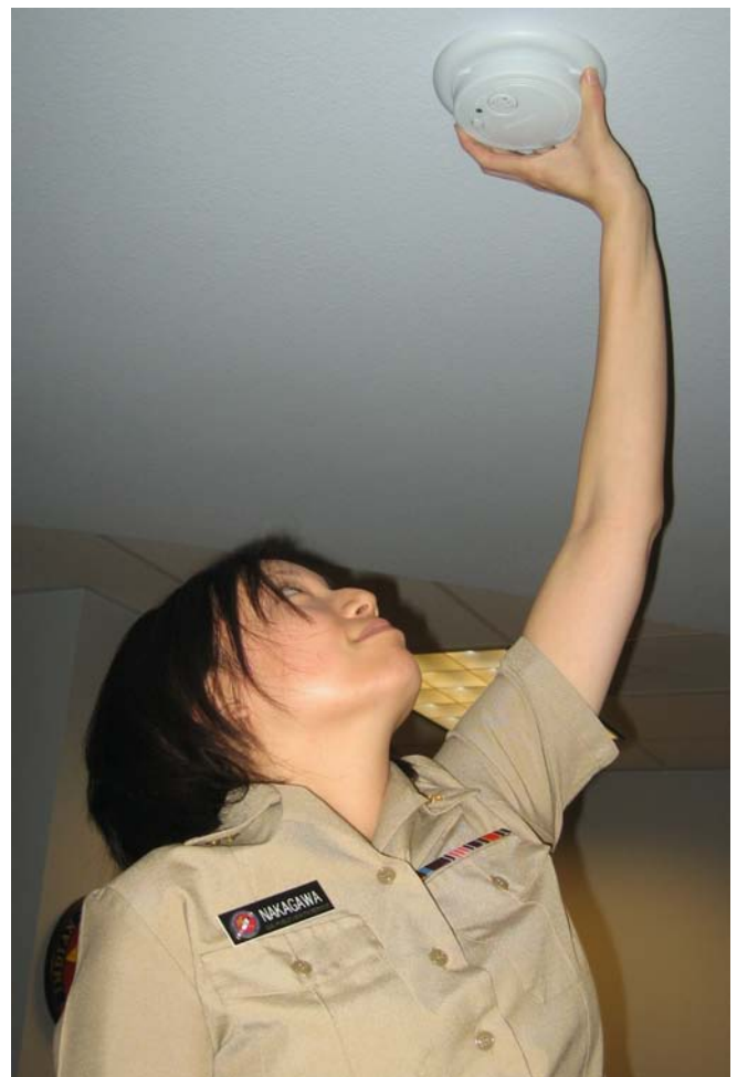
Area Injury Prevention Specialist, Lisa Nakagawa, installing a smoke detector in a residential home.
