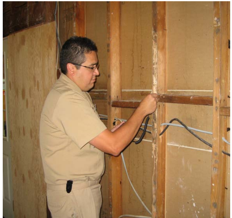
LCDR Martin Smith tests the moisture content in a Tribal facility as part of a mold assessment
