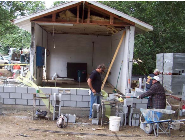
Pumphouse construction at United Indian Health Center, Inc. (Smith River, CA)
