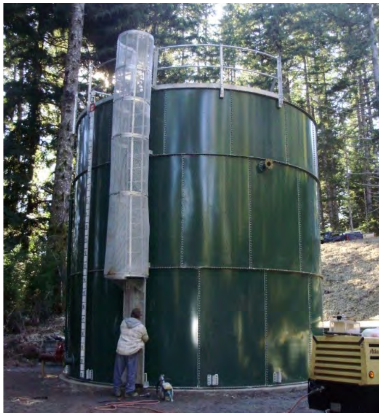
Water storage tank
