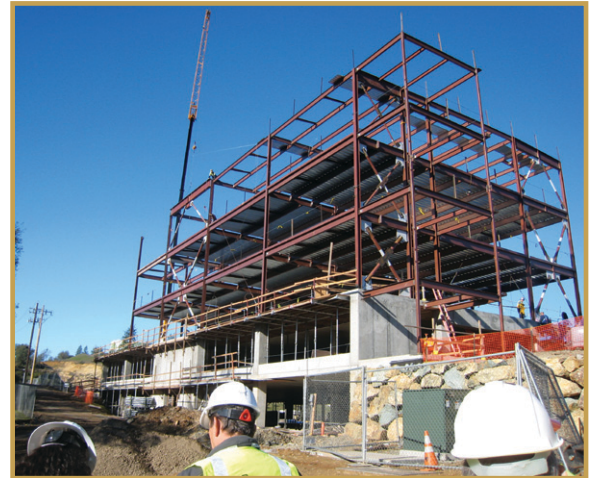
Shingle Springs Health & Wellness Center under construction. Below: DHFE employees inspect the Yuba City Clinic remodel.
