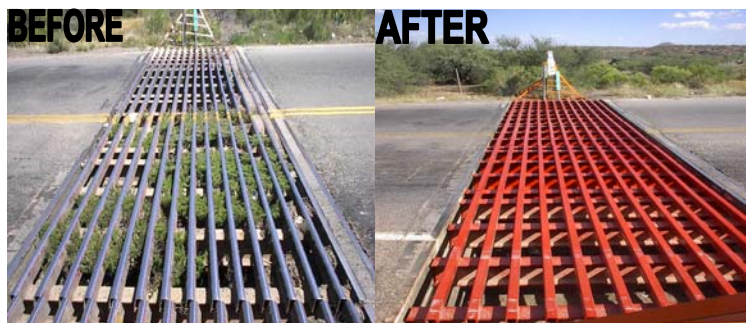
The San Carlos Apache Tribe received $50,000 to replace/repair defective cattle guards in an attempt to reduce livestock related crashes.
