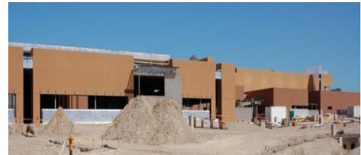
Figure 1 - San Carlos facility under construction
