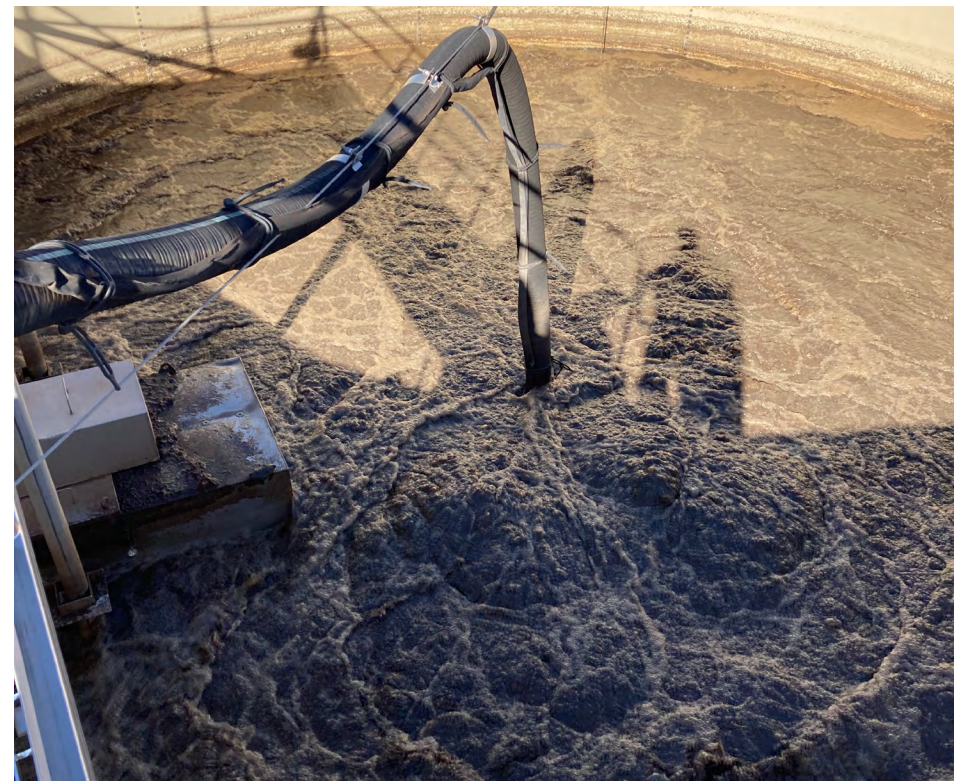
Wastewater undergoing aeration process.
