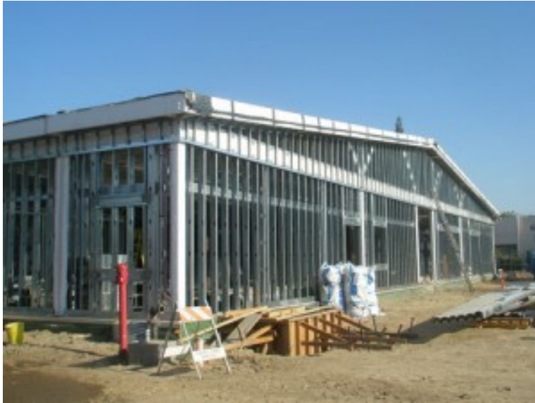
Facility 3 - Sierra Kings District Hospital, Reedley CA
