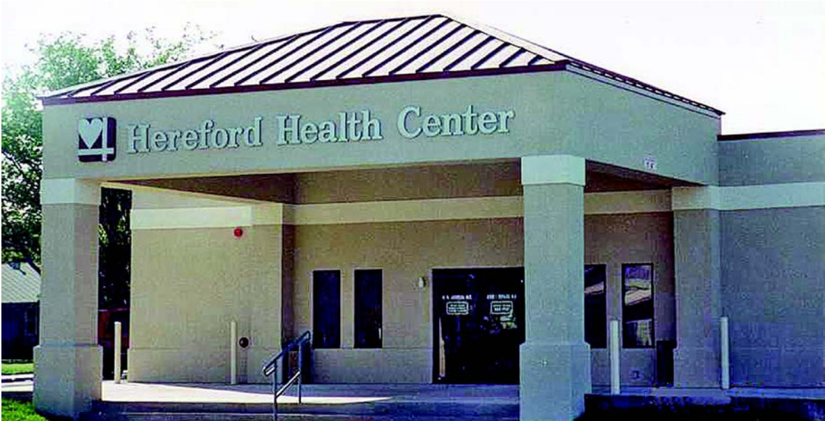
Facility 2 - Hereford Health Center, Hereford, TX
