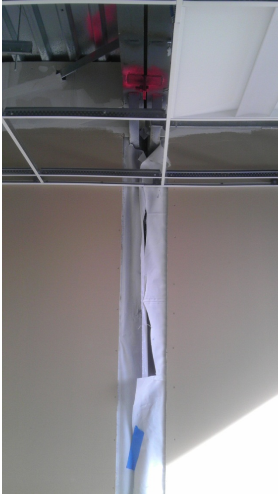
Cut Wall and Ceiling
