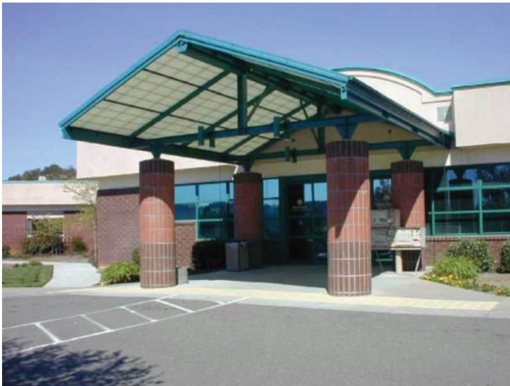
Facility 4 - Healdsburg General Hospital, Healdsburg CA
