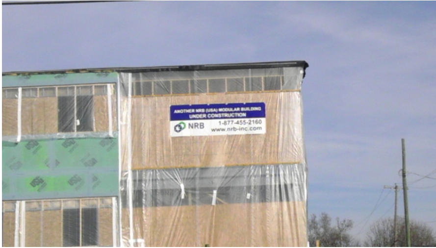
Modules After Initial Framing
