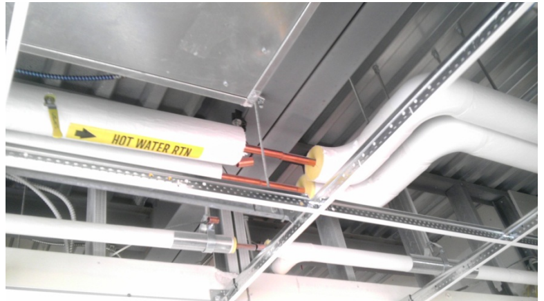
Cut Wall, Ceiling, and Piping
