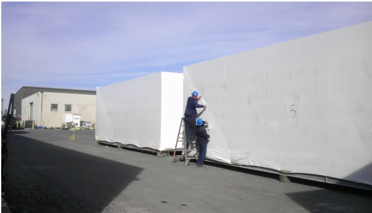
Modules Wrapped and Ready for Transport
