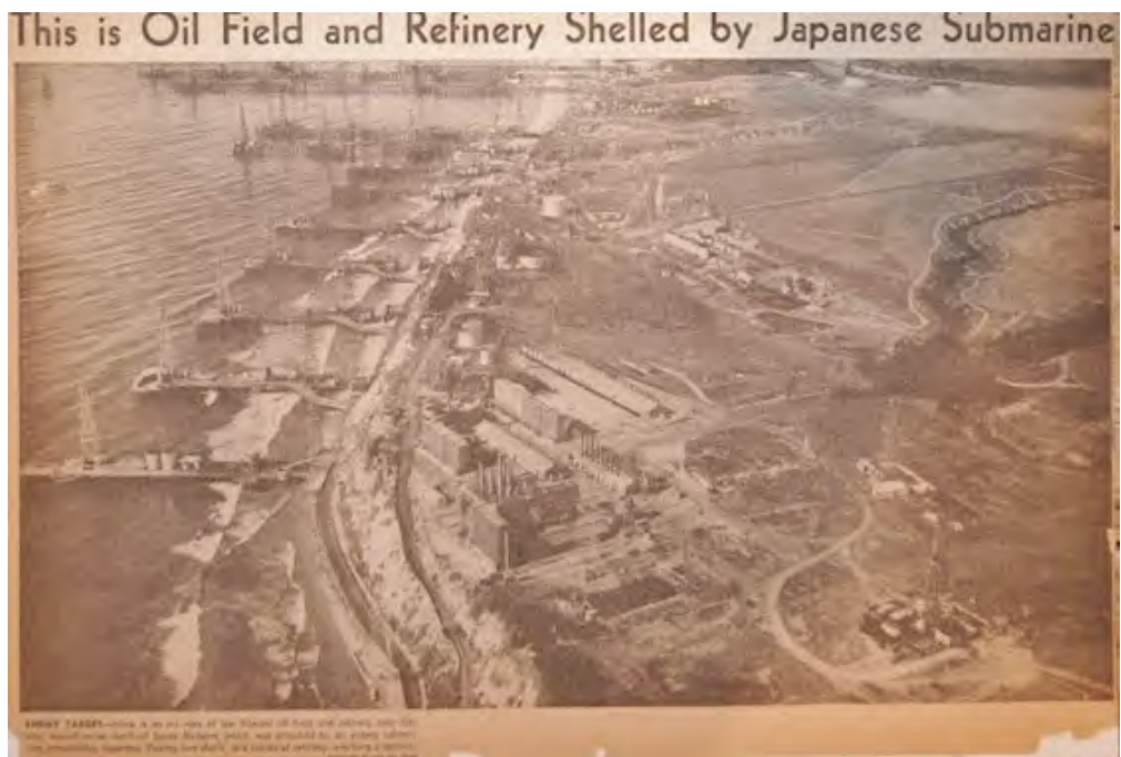
Figure 6. Bankline Oil Refinery after shelling on February 24, 1942
