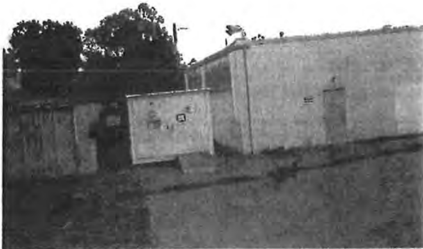
East façade and portion of north façade of shop, view southeast, 2-27-06, SBCo-FH-05-5037-035.jpg
