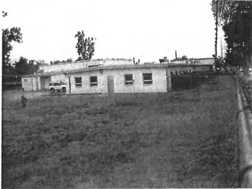
East façade of hall with assembly hall in background, view west, 2-27-06, SBCo-FH-05-5037-038.jpg
