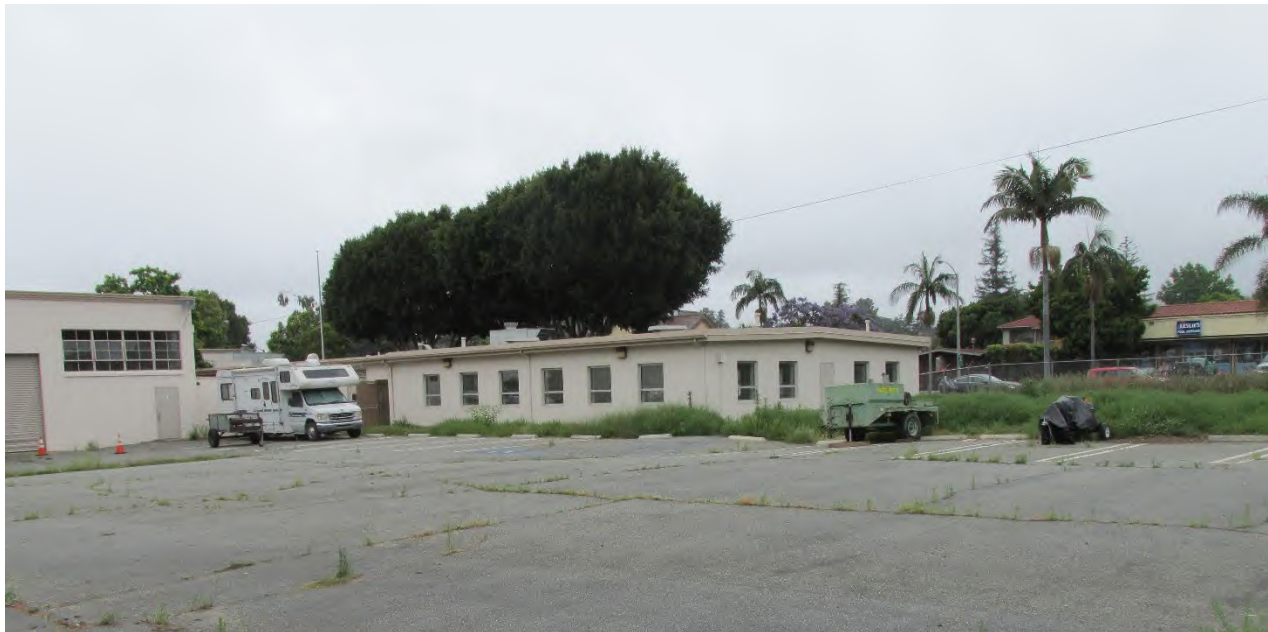
Figure 3. Assembly Hall addition on south elevation of Fremont Hall USAR Center looking northwest. (IMG_8360)
