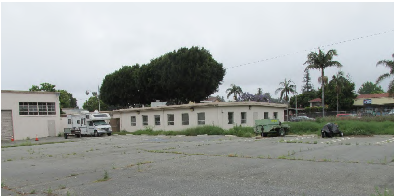
Figure 11. Assembly Hall addition on south elevation of Fremont Hall USAR Center, looking northwest. (IMG_8360)
