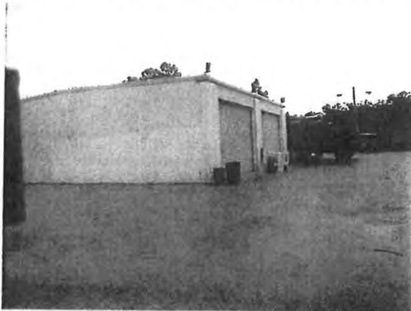
North and west façades of OMSA shop, view southeast, 2-27-06, SBCo-FH-05-5037-037.jpg
