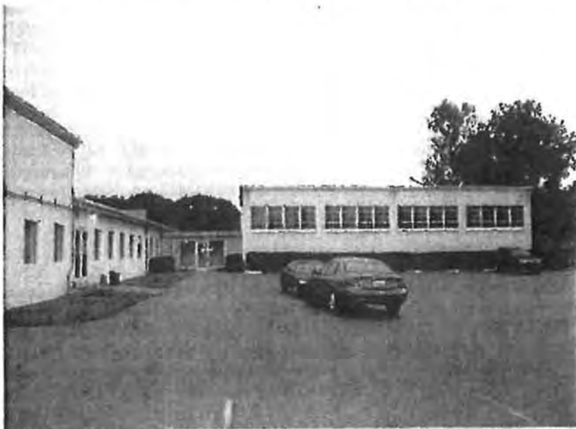
Rear of center and east façade of assembly hall, view east, 2-27-06, SBCo-FH-05-5037-027.jpg
