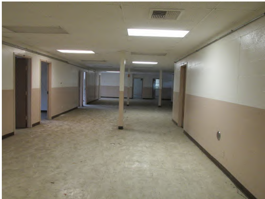
Figure 5. Interior of Fremont Hall USAR Center, looking west. (IMG_8378)
