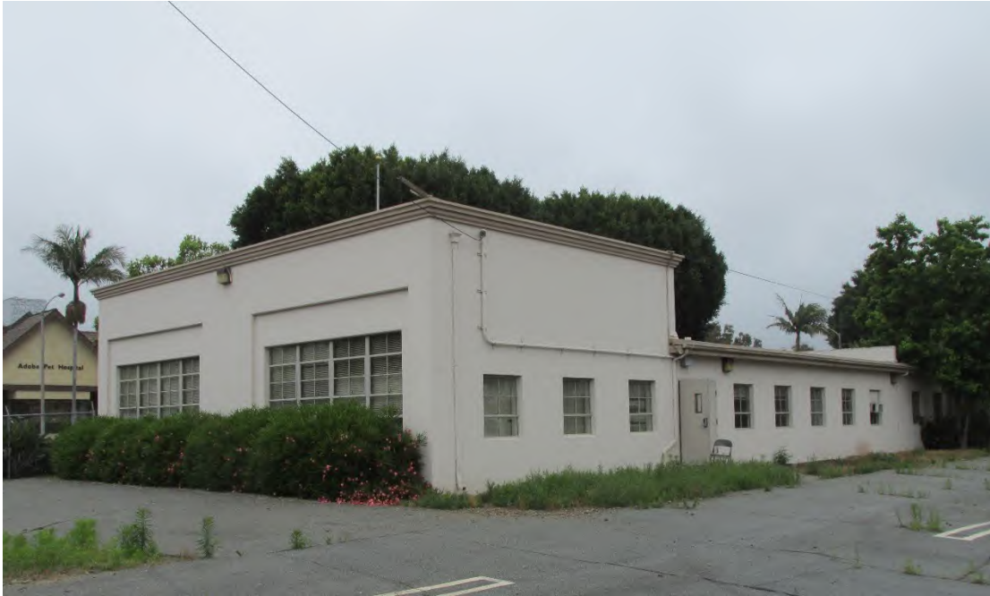
Figure 10. West elevation of Fremont Hall USAR Center, looking northeast. (IMG_8413)
