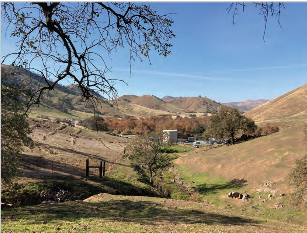
Drain fields left, WWTP center, new spray fields right, looking northwest (western edge of BLM land)
