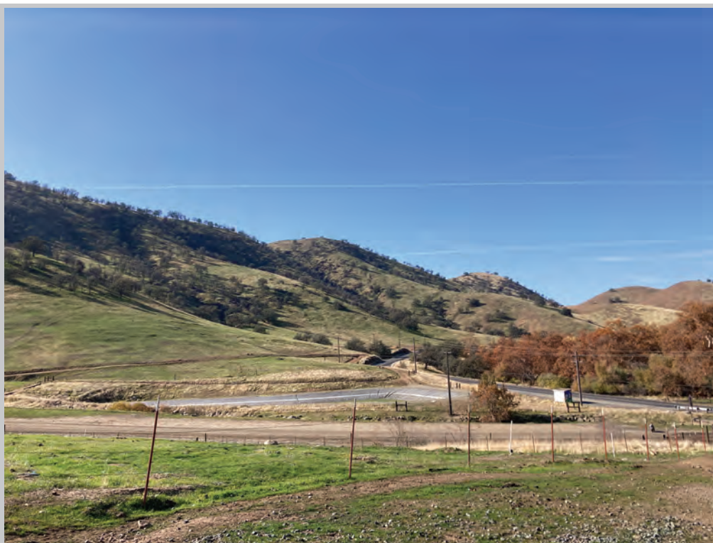
Existing untreated wastewater emergency storage pond
