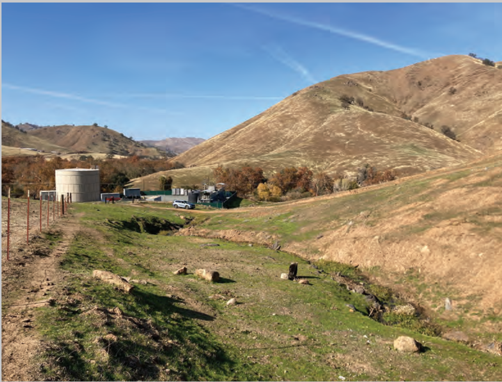
WWTP, location of future 900,000 gallon tank (behind existing tank), looking northwest
