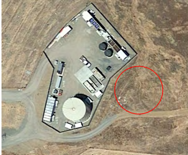
Figure 6: Storage Tank Location
