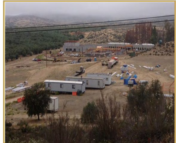
Above: Desert Sage Healing Center, Under Construction, Hemet, CA
