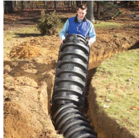
Infiltrator chambers can be installed in curved, sloped and small areas allowing for optimal land use.
