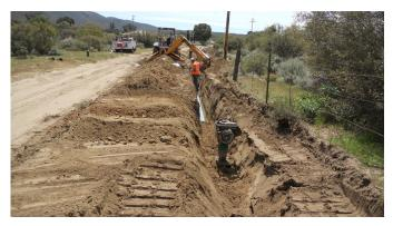
Water Main Construction on the Santa Rosa Reservation Utilizing \$1.1 million in U.S. Department of Agriculture, Rural Development funding, the SFC program worked with the Santa Rosa Tribal Government to construct approximately five miles of water mains (4, 6, and 8 inch pipelines), installed metered water service connections, and drilled/equipped a new community drinking water well under IHS Project CA 09-Y04. This project served over 40 tribal homes and offices.
