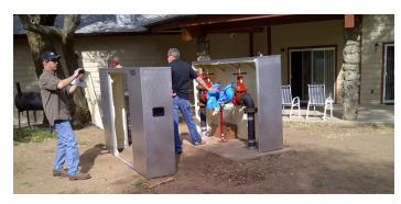
A backflow prevention assembly being installed for the Tribal Hall fire sprinkler protection system has a heated enclosure to protect from below freezing temperatures
