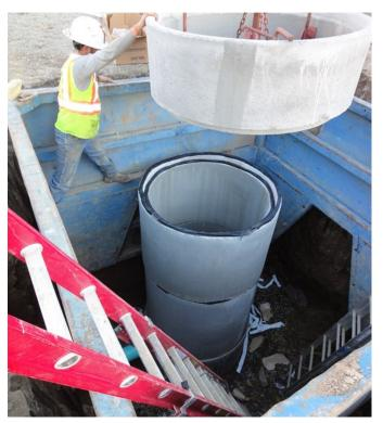
Installing 6-foot diameter concrete sections—Sewage Lift Station
