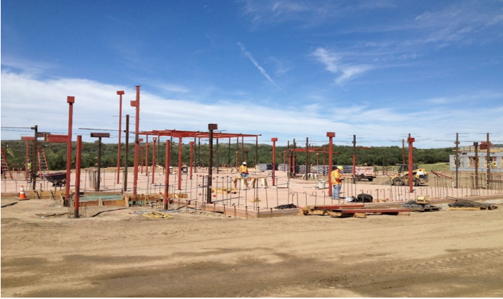
Desert Sage Youth Wellness Center Structural steel construction
