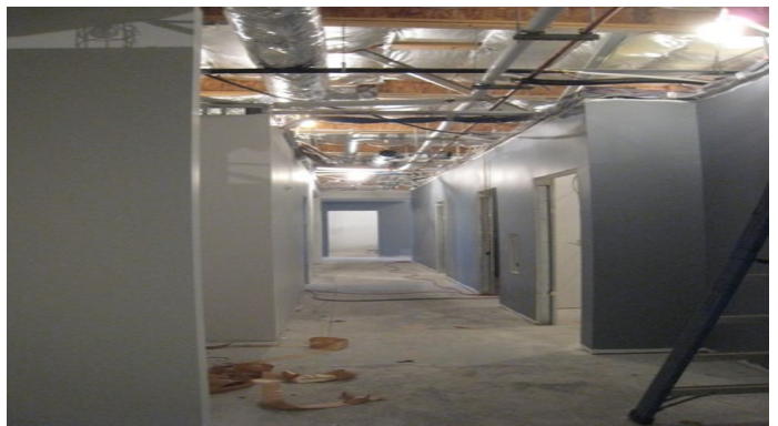
Lake County Tribal Health Consortium Lakeport OB & Peds Clinic remodel
