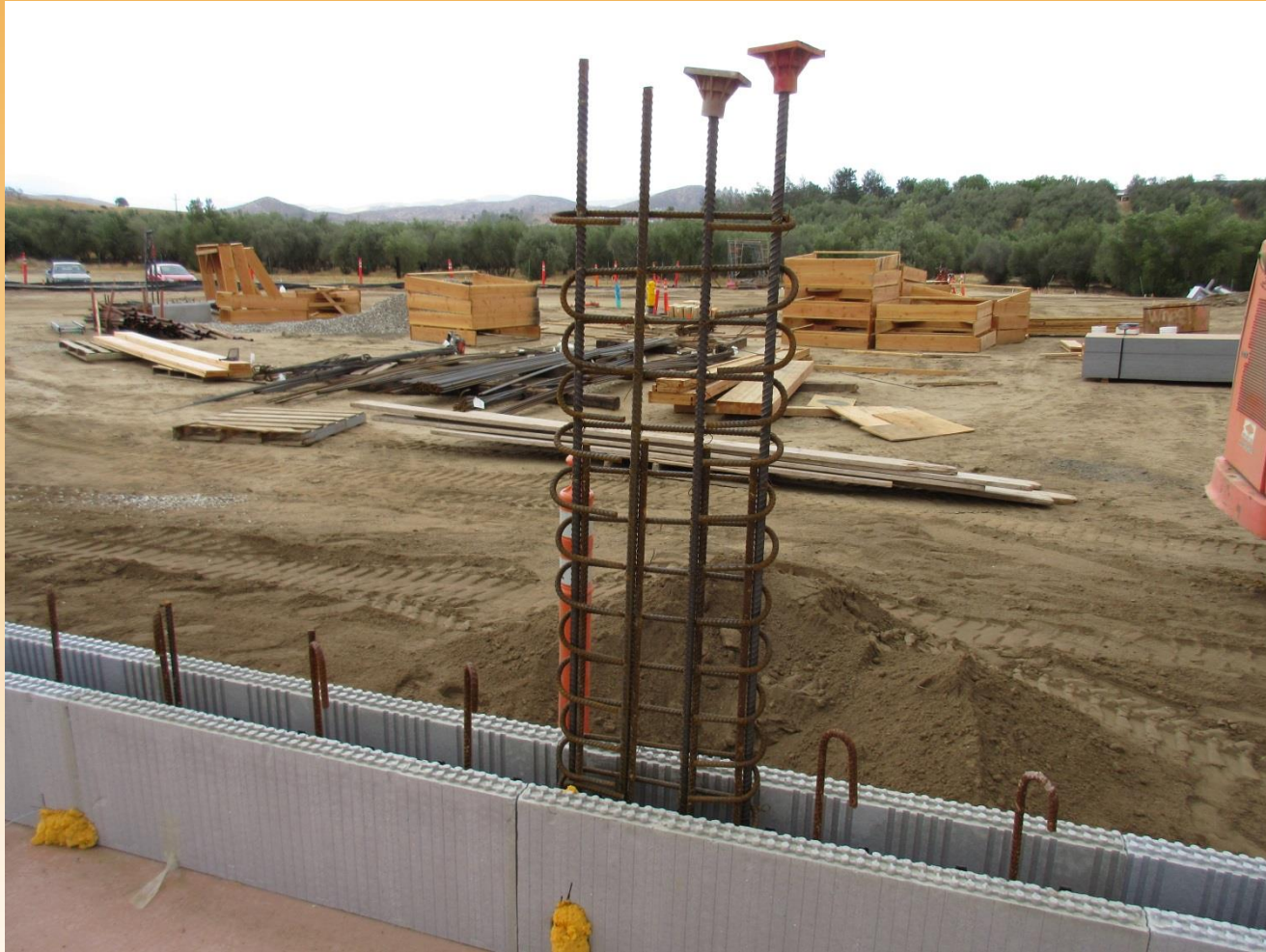
Example - Insulated concrete filled (ICF) wall
