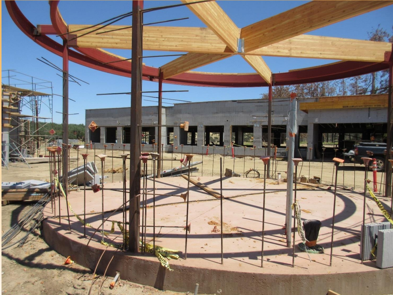
Cultural Building (E) – Structural Steel, Glulam Beams, Rebar
