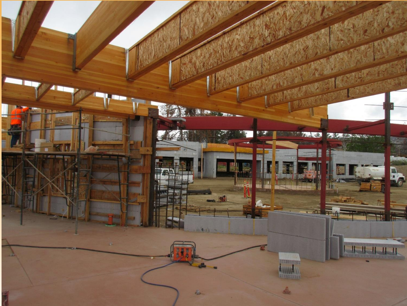
Admin/Therapy Building (C) – Glulam Beams, Joists, & ICF Walls
