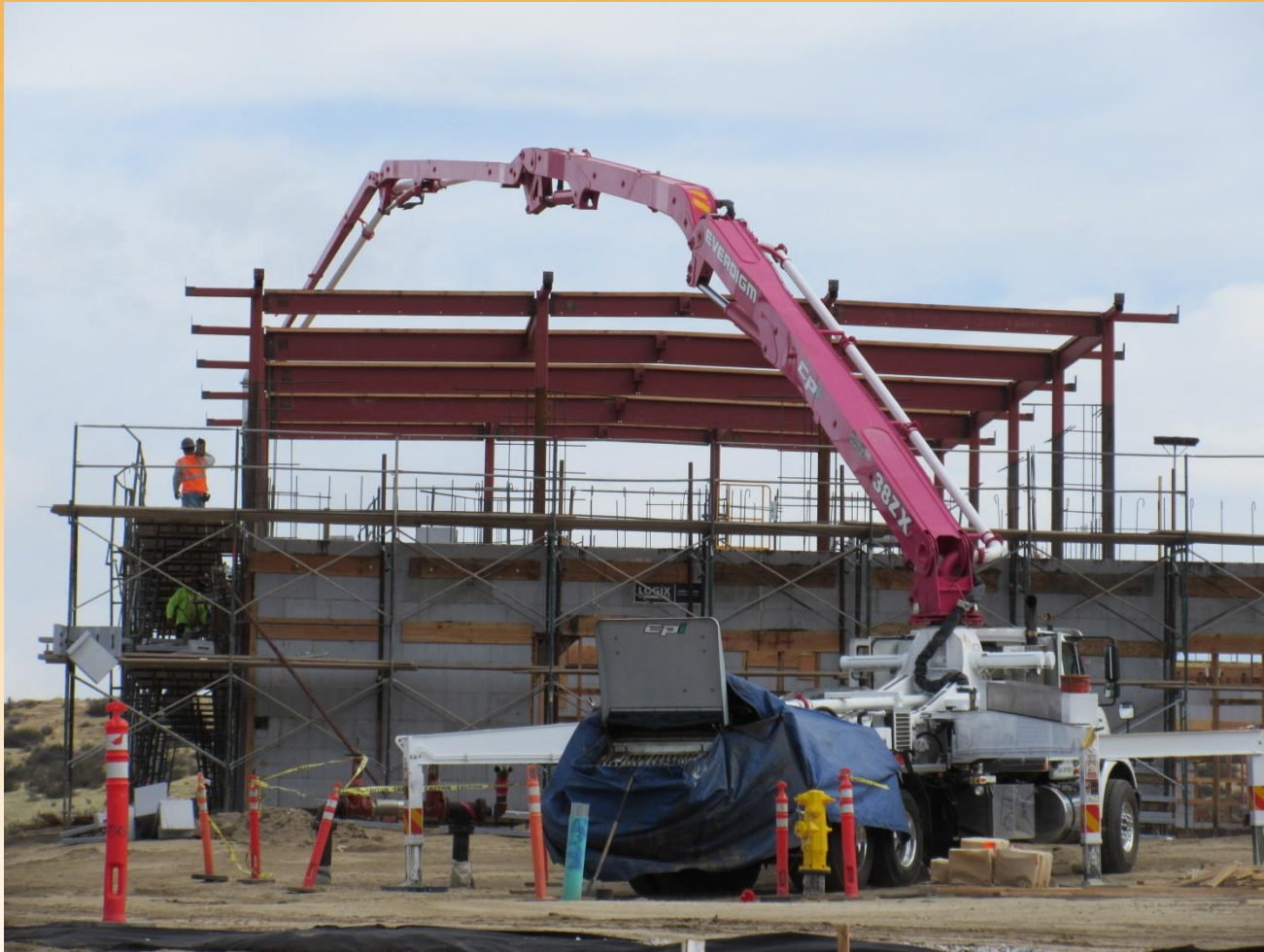
Gymnasium (B) – Pumping concrete to ICF Wall
