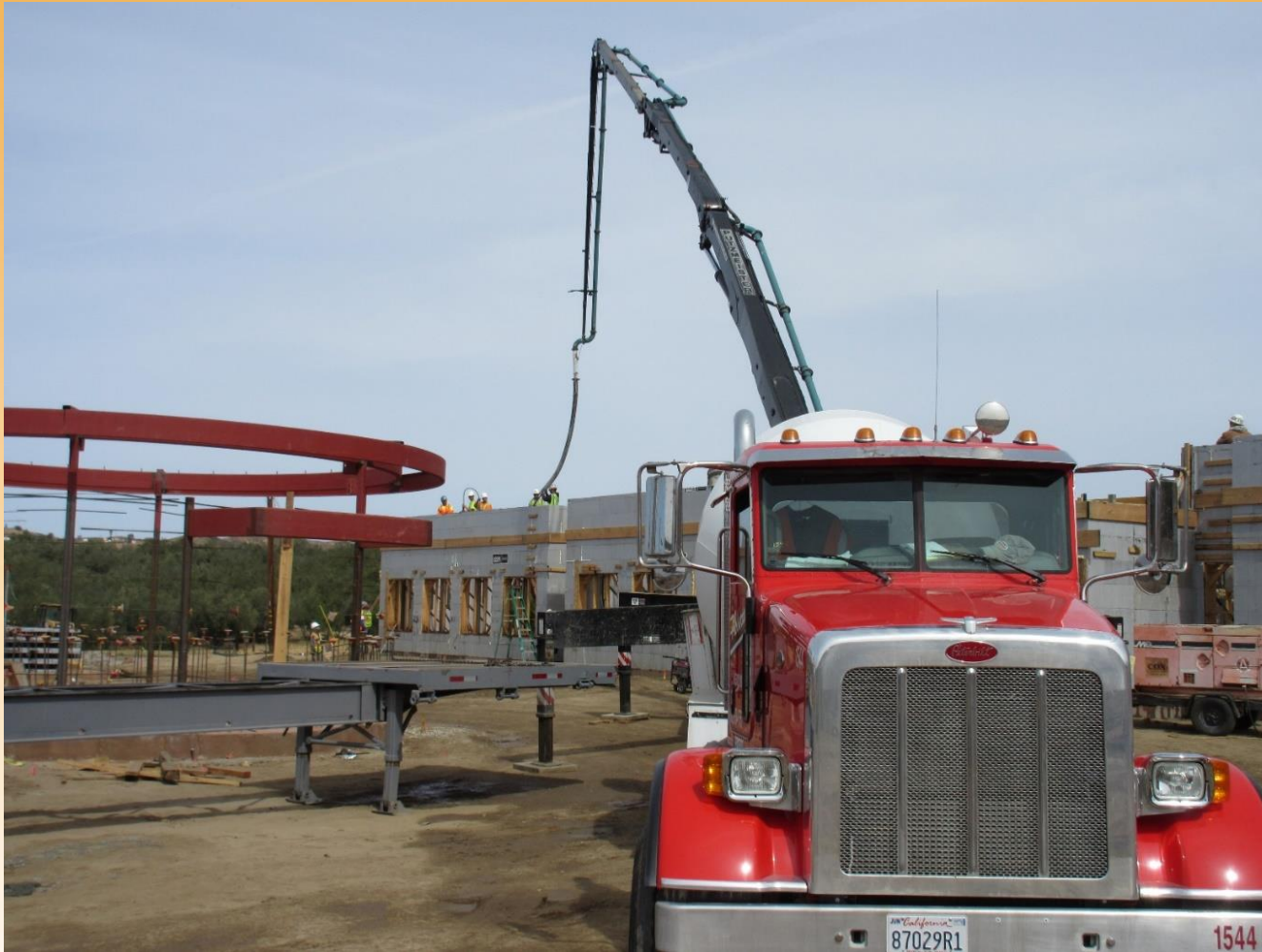
Resident Building (A) – Placing concrete in ICF wall
