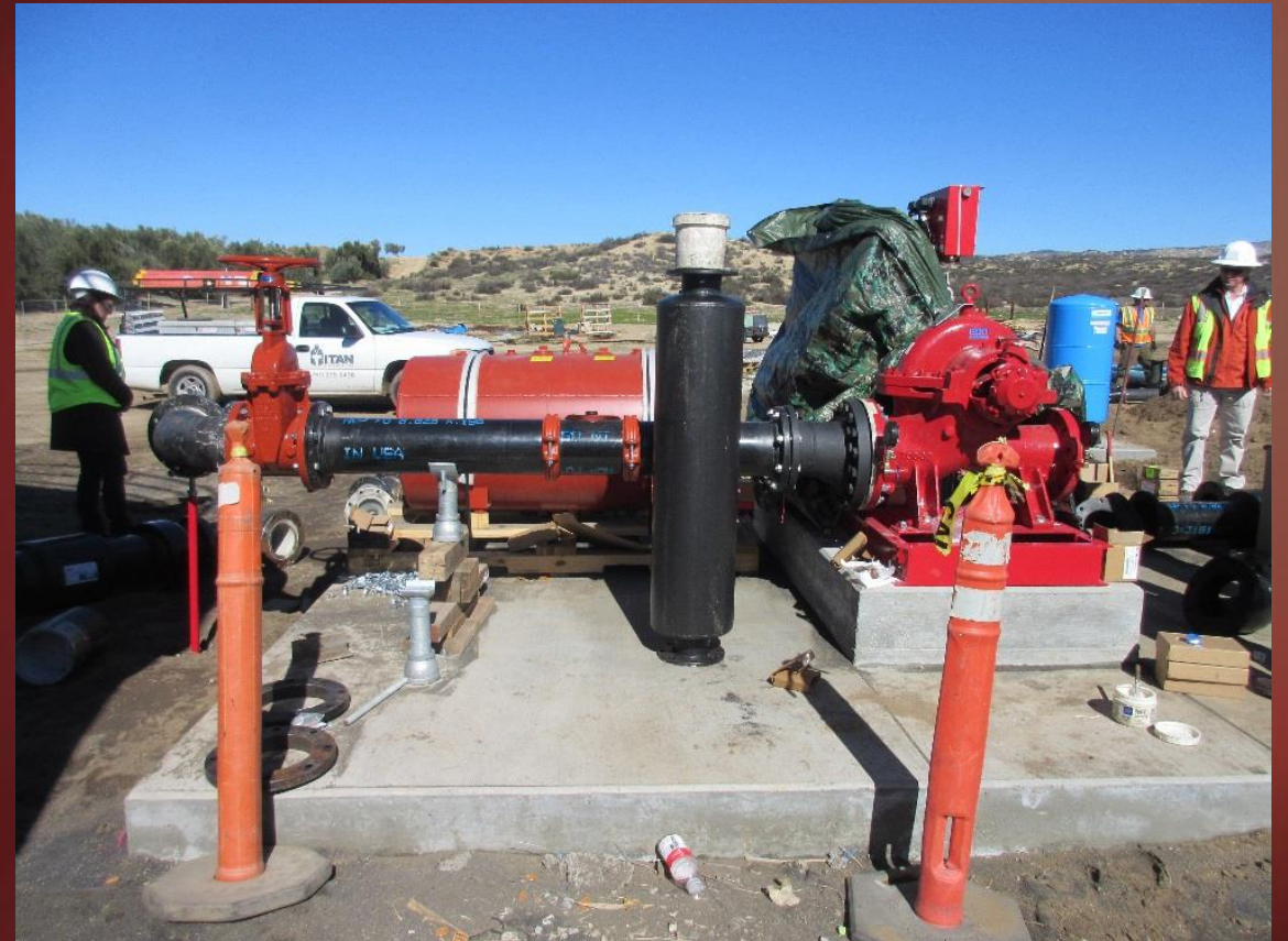
Well Pump Installation
