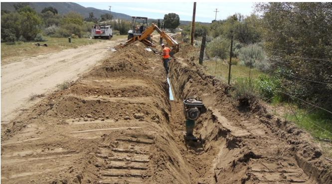
Water Main Construction on the Santa Rosa Reservation Utilizing \$1.1 million in U.S. Department of Agriculture, Rural Development funding, the SFC program worked with the Santa Rosa Tribal Government to construct approximately five miles of water mains (4, 6, and 8 inch pipelines), installed metered water service connections, and drilled/equipped a new community drinking water well under IHS Project CA 09-Y04. This project served over 40 tribal homes and offices.
