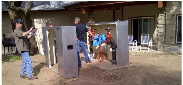
A backflow prevention assembly being installed for the Tribal Hall fire sprinkler protection system has a heated enclosure to protect from below freezing temperatures
