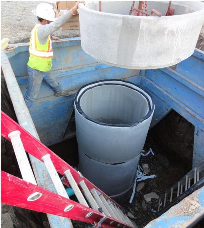
Installing 6-foot diameter concrete sections—Sewage Lift Station
