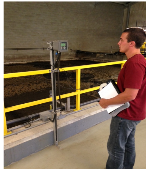
Inspecting Sequence Batch Reactor at a Wastewater Treatment plant
