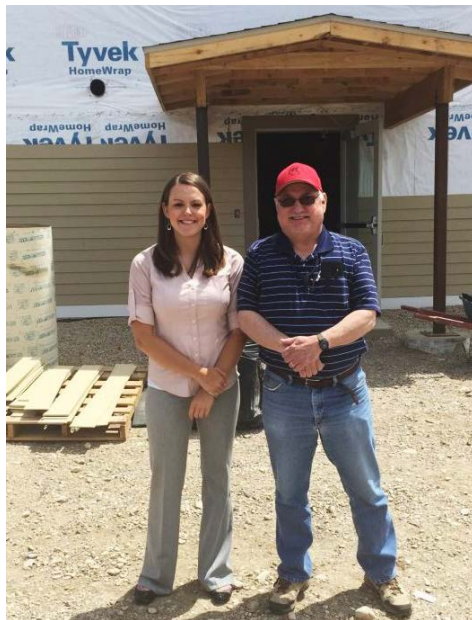
Environmental Health Officer Jim Dodd and I at a construction site on the Turtle Mountain Reservation
