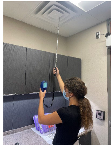
Measuring air flow in an Indian clinic with a VelociCalc ventilation meter
