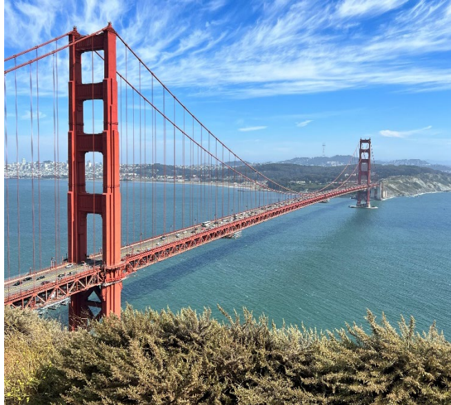
Picture of Golden Gate Bridge from travels to San Francisco
