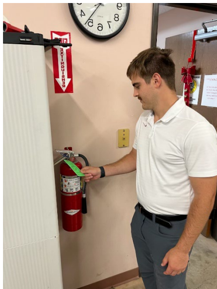
Inspecting a portable fire extinguisher
