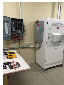
Fig. 1. Power Logger (Fluke 1735) installed in the output of the Inverter
