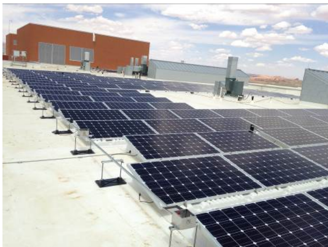
Fig. 3: Kayenta PV System
