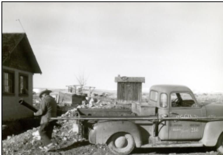
Figure 1: Construction of a septic system, 1960's
