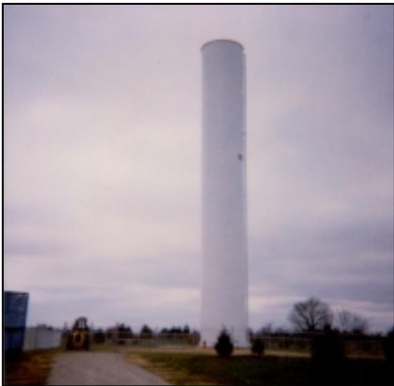
**Figure 13:** Completed 16' x110', 60,000 gallon stand pipe.
