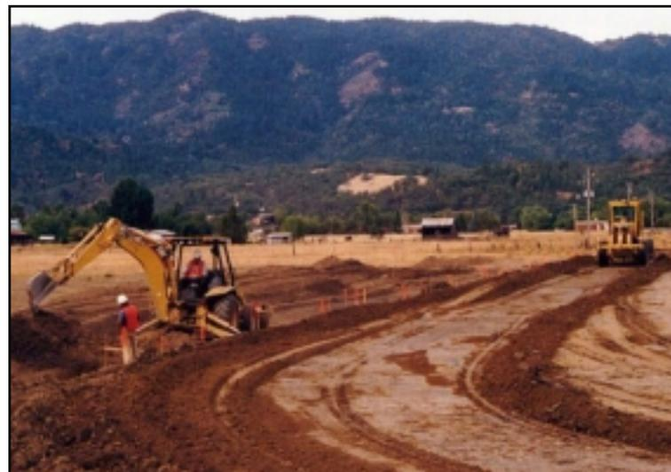
**Figure 21:** Construction of the south dike of the AIWPS outer treatment pond cell
