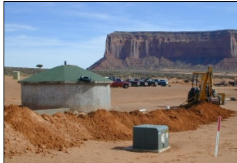
**Figure 25:** Bathroom addition and waterline construction at a hogan in Monument Valley, AZ.
