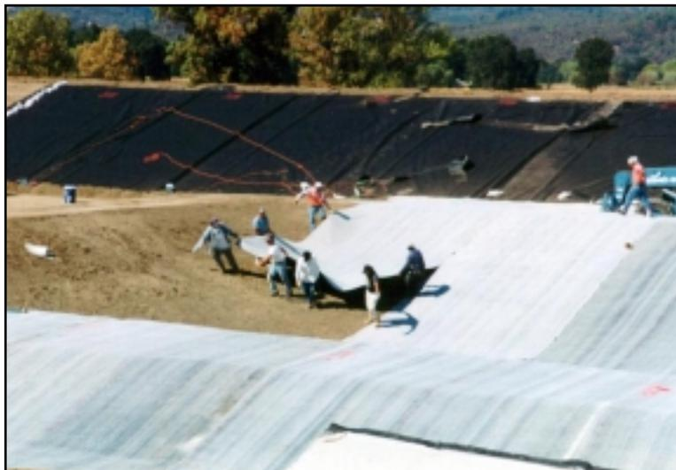
**Figure 22:** Installation of the Reinforced Geosynthetic Clay Liner(GCL) in the AIWPS Fermentation Cell Pit.
