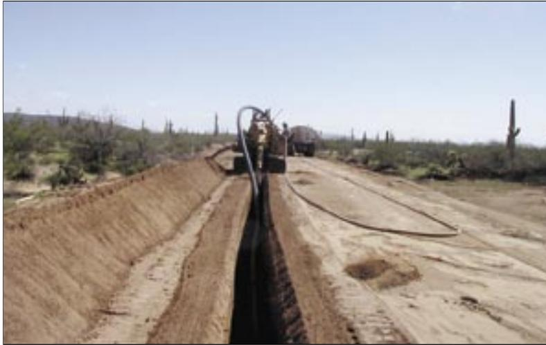
**Figure 23:** Laying HDPE pipe.
