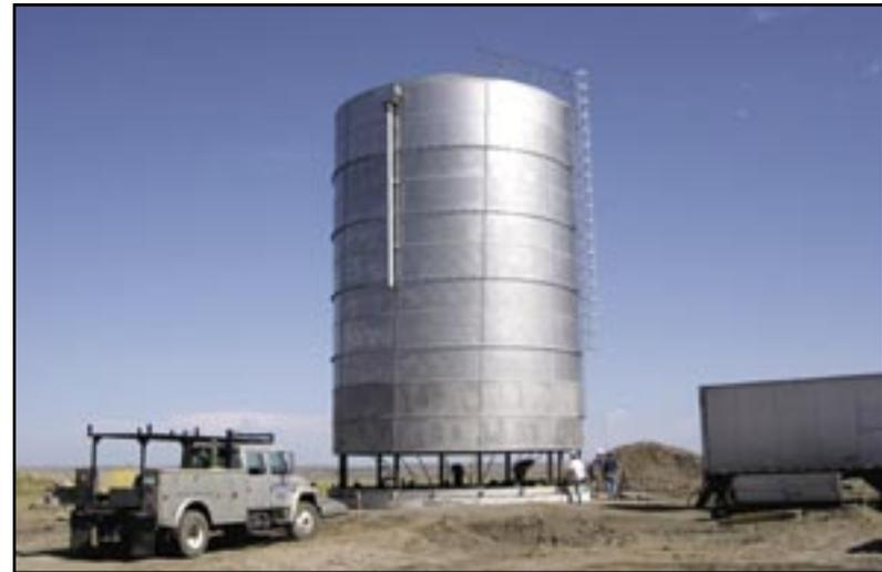
Figure 10: New 300,000-gallon stainless steel reservoir.
