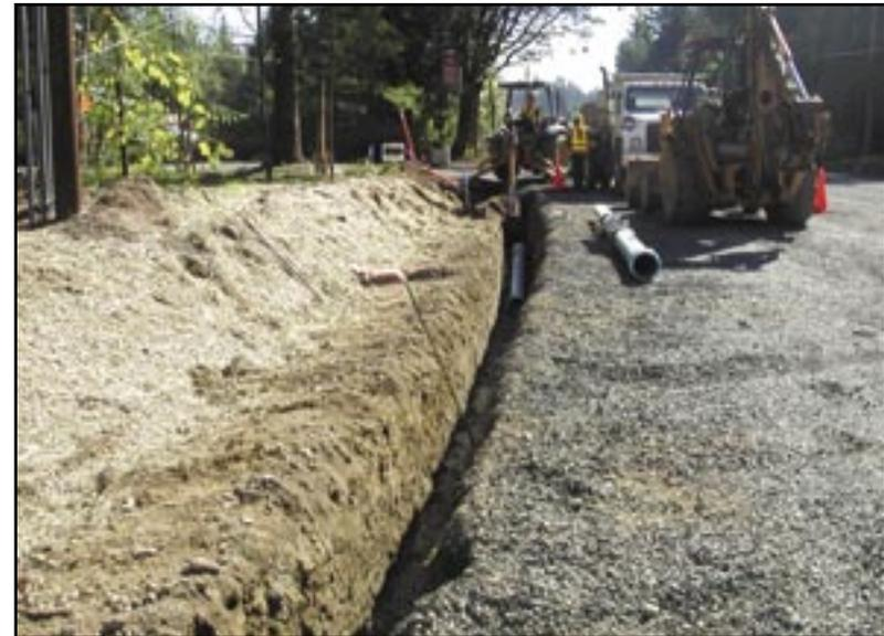
Figure 29: 8" PVC water main installation.
