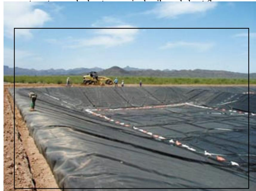
Figure 19: Anchor trench installation.
