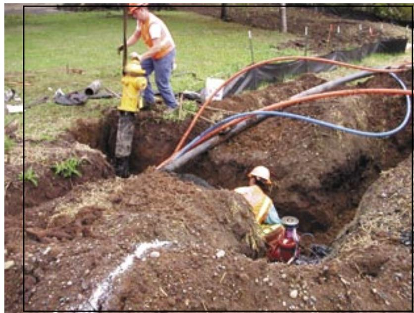
Figure 26: Hydrant installation.
