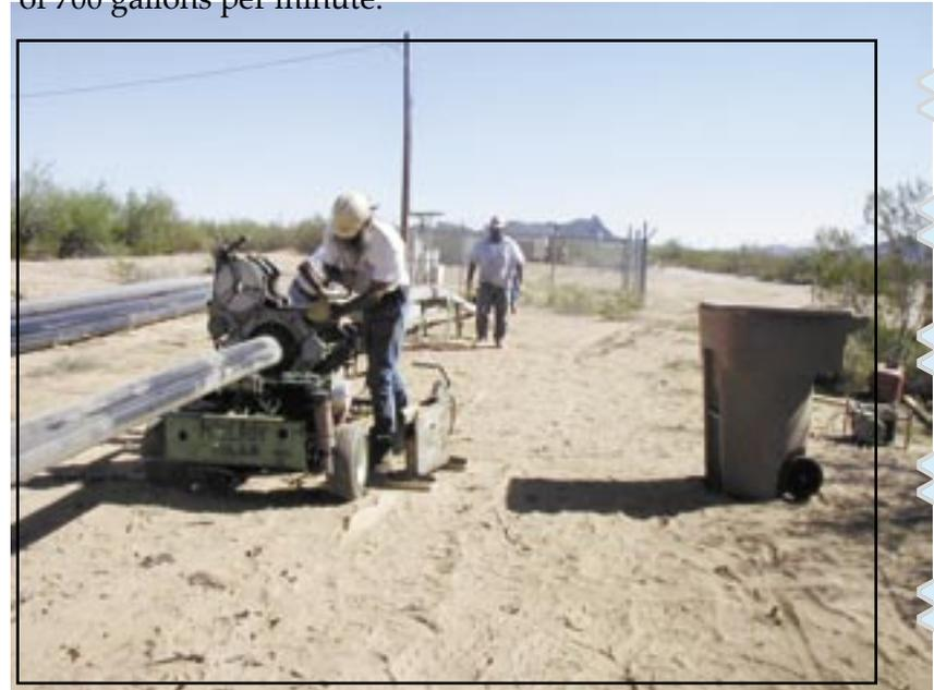
Figure 22: Fusing HDPE pipe.
