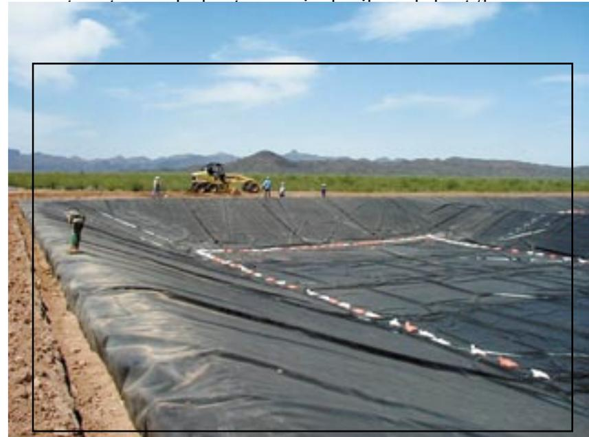
Figure 19: Anchor trench installation.
