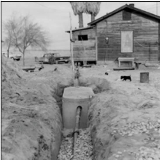
**Figure 1:** Construction of a septic system, 1960's.
