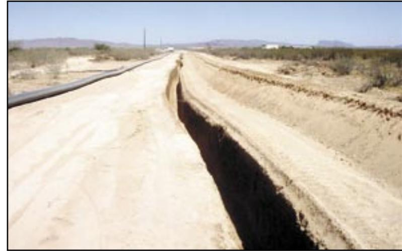
**Figure 24:** Sewerline trench.
