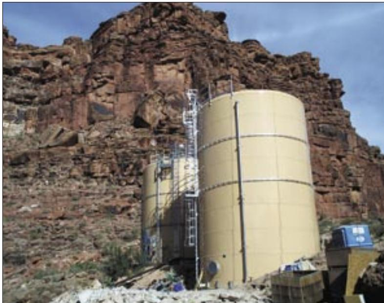
Figure 16: New 108,000-gallon water storage reservoir.
