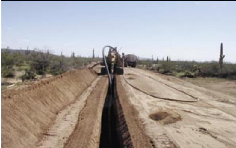
**Figure 23:** Laying HDPE pipe.
