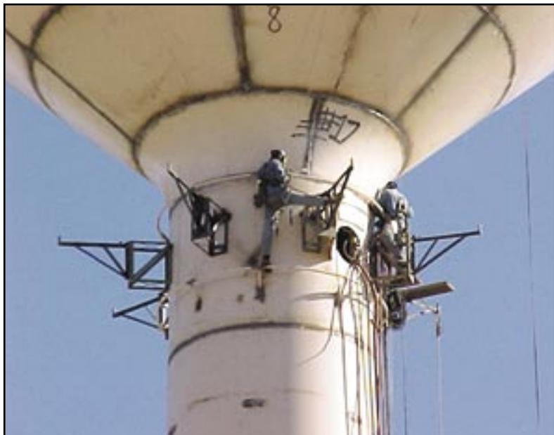
Figure 37: Welding on a watersphere in Cocopah, Arizona
