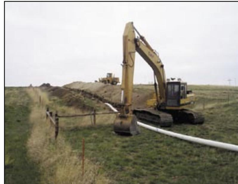
**Figure 11:** Waterline installation.
