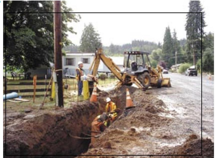
Figure 28: 8" PVC water main installation.
