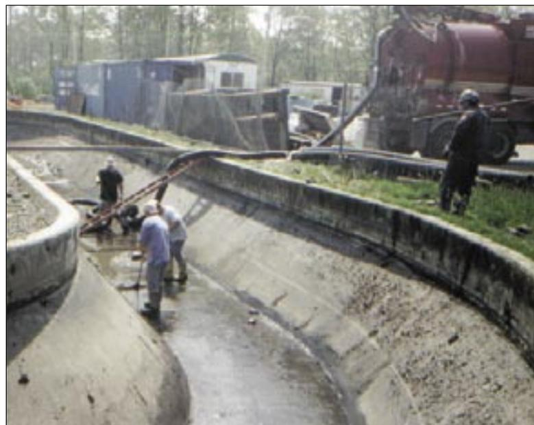
**Figure 8:** Cleaning an oxidation ditch in Penobscot, Maine.
