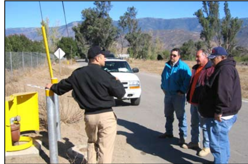
Figure 21: IHS engineer explains an air vacuum release valve to tribal representatives during a final inspection.
