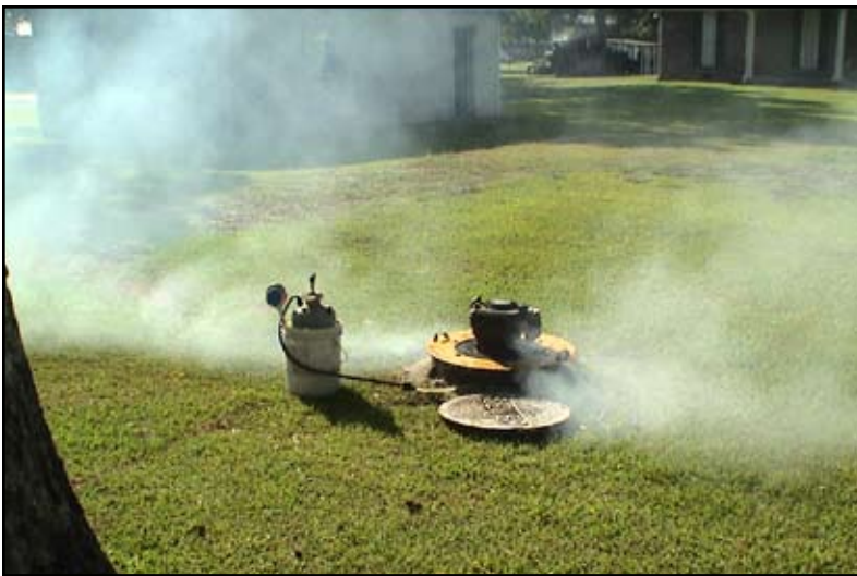
Figure 24: Smoke testing sewer mains at Chitimacha Reservation.
