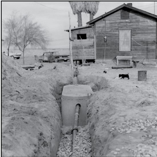
Figure 1: Construction of a septic system, 1960's.
