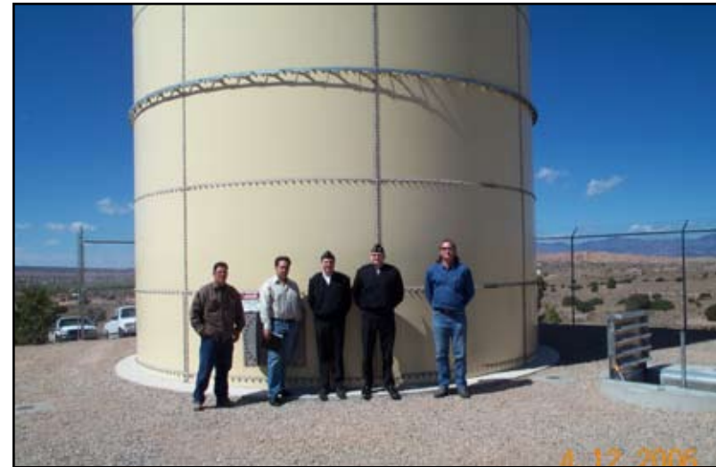
Figure 8: Water storage tank final inspection in Pojoaque Pueblo, NM.
