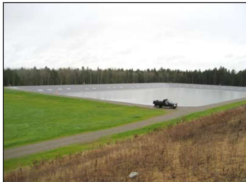
Figure 30: Completed 13 million gallon sewage lagoon for Passamaquoddy Tribe.
