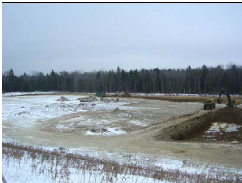
Figure 29: Construction of sewage lagoon expansion for Passamaquoddy Tribe.
