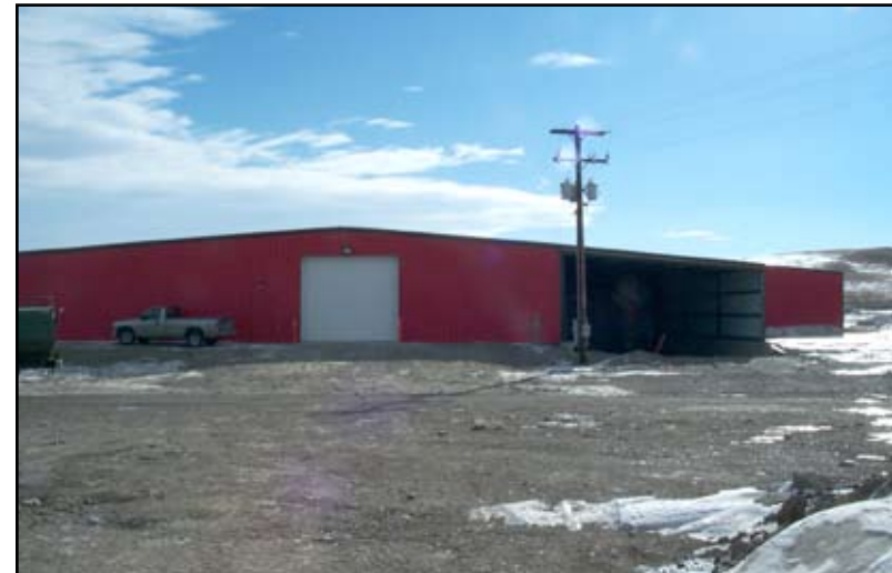
Figure 10: Lumber mill building was remodeled to become the solid waste transfer site.
