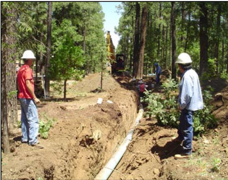
Figure 4: COSTEP Stephen Irwin and IHS inspectors Manual Quesada and Ron Burnette discuss maximum allowable pipe deflection on Fort Apache Indian Reservation, Hon Dah, Arizona.
