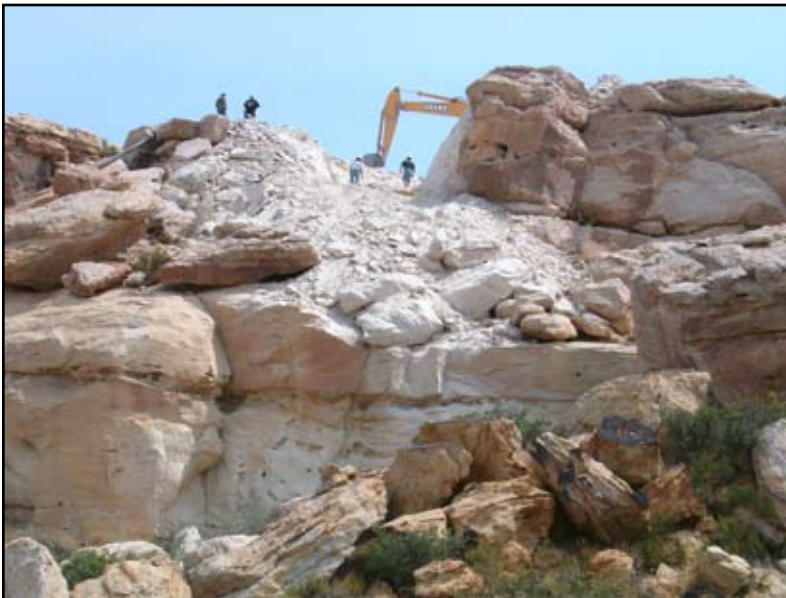
Figure 31: Construction of sewer outfall line for Village of Shungopavi, Hopi Reservation.
