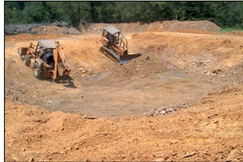
Figure 13: Okmulgee crew sloping an individual wastewater lagoon.
