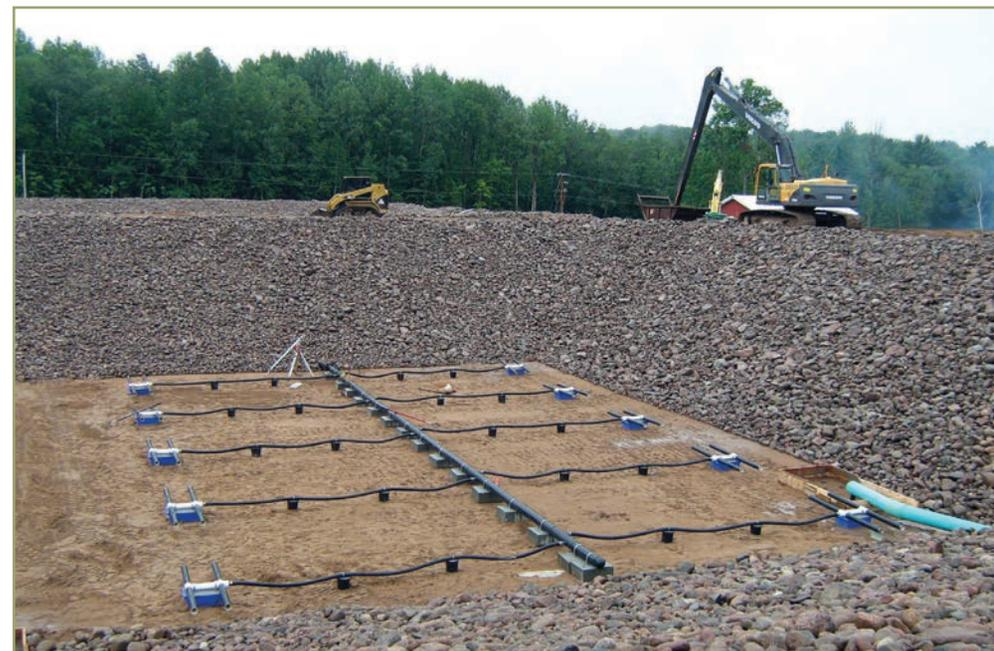
Completion of the ET system which disposes of wastewater into the atmosphere through evaporation.
