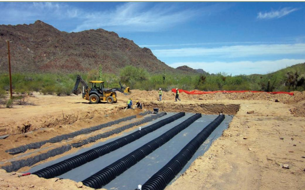
Construction of a Evapo-transpiration (ET) sand bed, Arizona.
