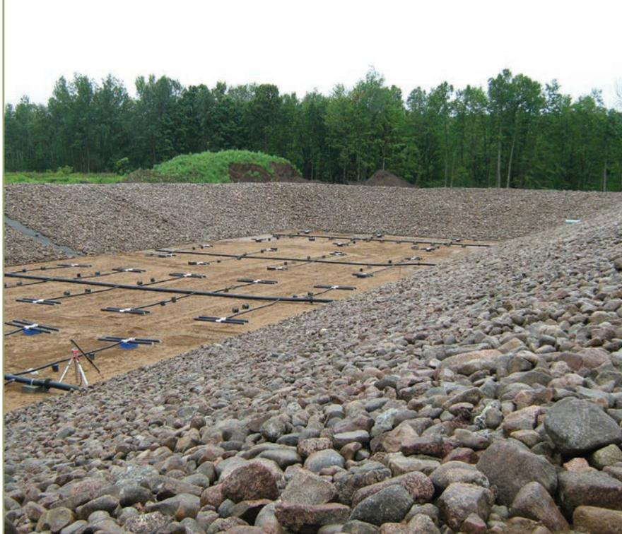
Installation of diffusers in the new aerated lagoon cell, Wisconsin.
