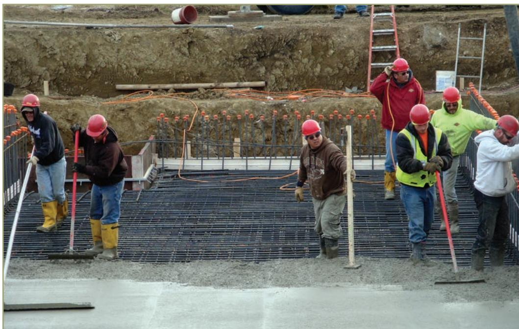
Contractor pouring the foundation for a 100k gallon buried concrete reservoir for on the Lake Traverse reservation, South Dakota.
