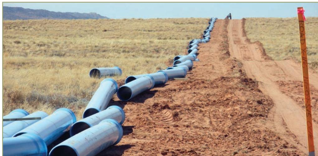
Construction of a 14" waterline located in Sweetwater on the Navajo Reservation.
