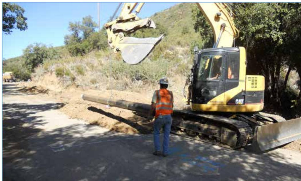
Water pipe in steel casing being installed at culvert crossing.
