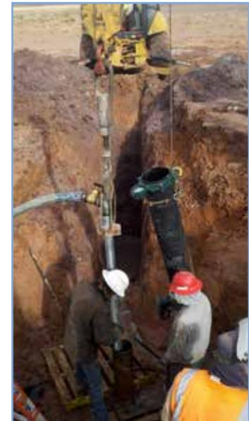
Installing pitless adapter on well casing, Utah.
