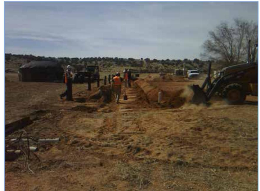
Installation of a septic tank/drainfield system, Arizona.
