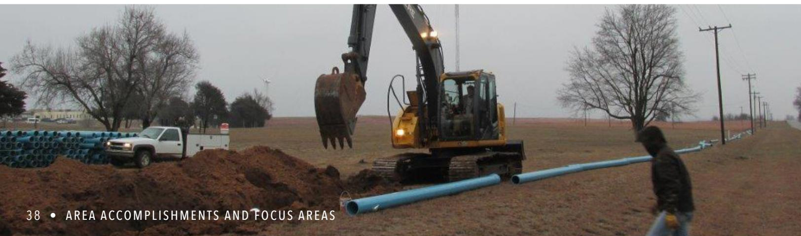
Additionally, Indian Health Service Emergency and Special project funding was used to serve 190 Cherokee Nation homes with an 8 inch water main replacement for the Cherokee Rural Water District #7 at the Baron Fork Creek crossing, southeast of Tahlequah, Oklahoma. An influx of rain caused flooding that destroyed the previous water line that bridged the Baron Fork Creek.
