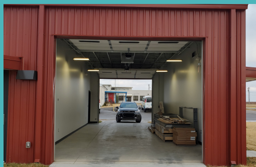
Kaw Nation's new loading dock for car seat installation.
