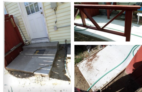
In Picture 1, stairs are visibly damaged, there are no handrails. Concrete is visible cracked and ground surrounding porch is uneven. Pictures 2 and 3 show the same home with new ramp and handrails.
