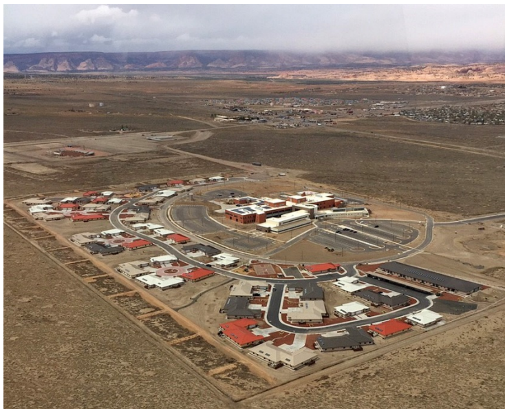
The newly constructed Kayenta Health Center / Alternative Rural Hospital in Kayenta, Ariz., will serve a population of more than 19,000 people.
