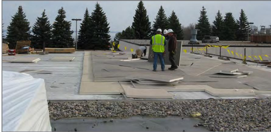
▲ Completion of a roof insulation project at Red Lake Hospital. This project was completed as an energy conservation measure project after being recommended in the audit process.
