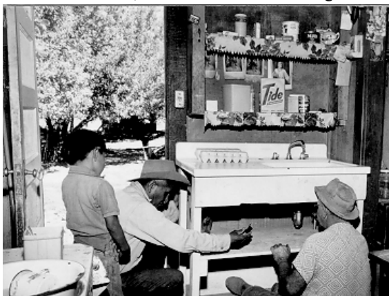
Figure 3-6. Installing a kitchen sink in an Indian home.
