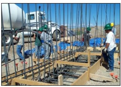
Figure 41: Tribal contractor preparing forms and reinforcement for solid waste transfer station at Taos Pueblo, NM
