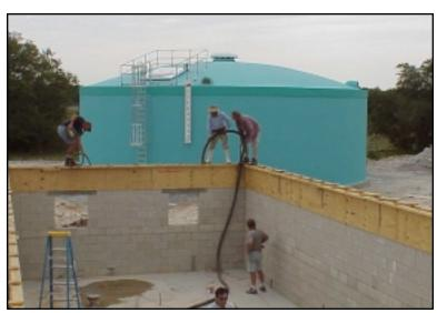
Figure 39: Construction of a pump station and ground level tank, Seminole Tribe, FL
