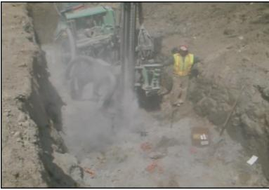
Figure 36: Drilling for rock removal to facilitate installation of water main, Bois Forte Reservation.
