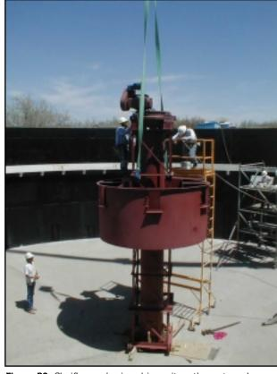
Figure 29: Clarifier mechanism drive unit on the center column.
