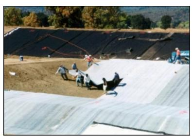
Figure 22: Installation of the Reinforced Geosynthethic Clay Liner(GCL) in the AIWPS Fermentation Cell Pit.
