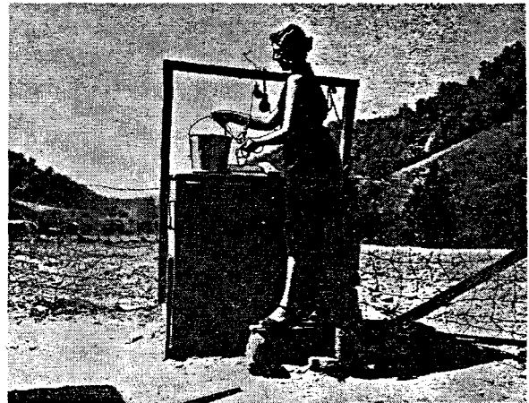
Typical dug well in group C area.
