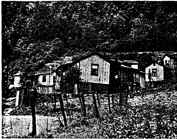
Representative housing in group C area.
