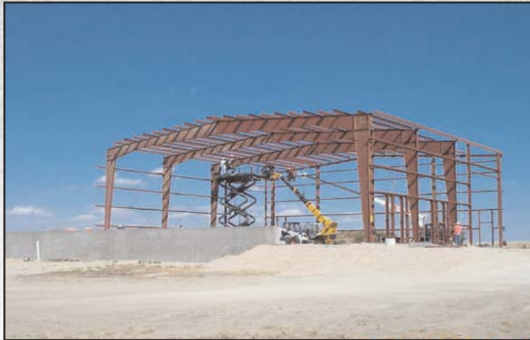
Figure 32: Skeleton of Pine Ridge Baler Building taking shape.
