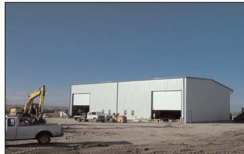
Figure 34: Completed Pine Ridge Baler Building
