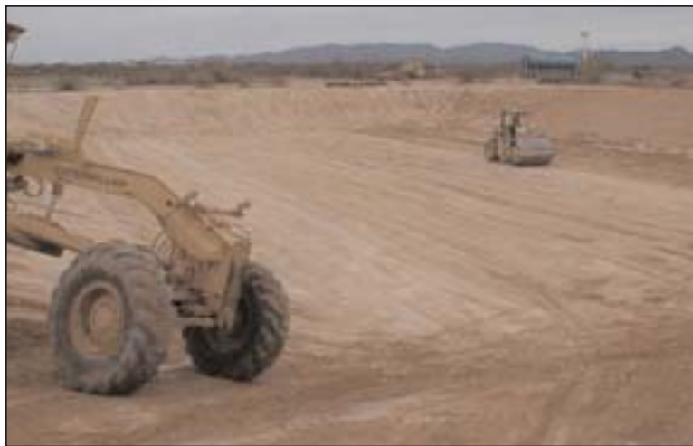
Figure 9: Construction of lagoon expansion cell.
