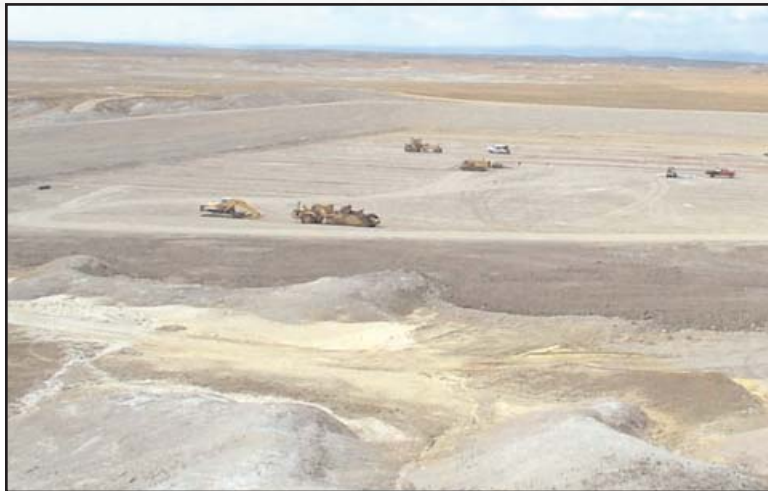
Figure 30: Construction of 10-acre landfill.
