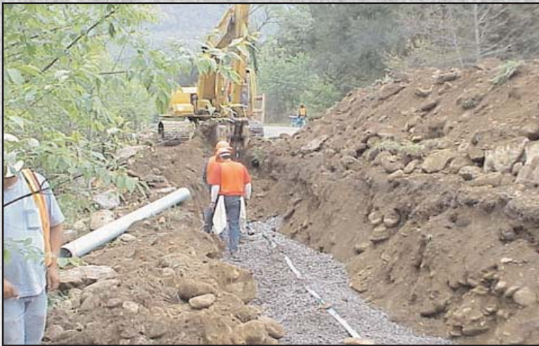
Figure 27: Big Cove Loop Road-8" PVC sewer lateral.
