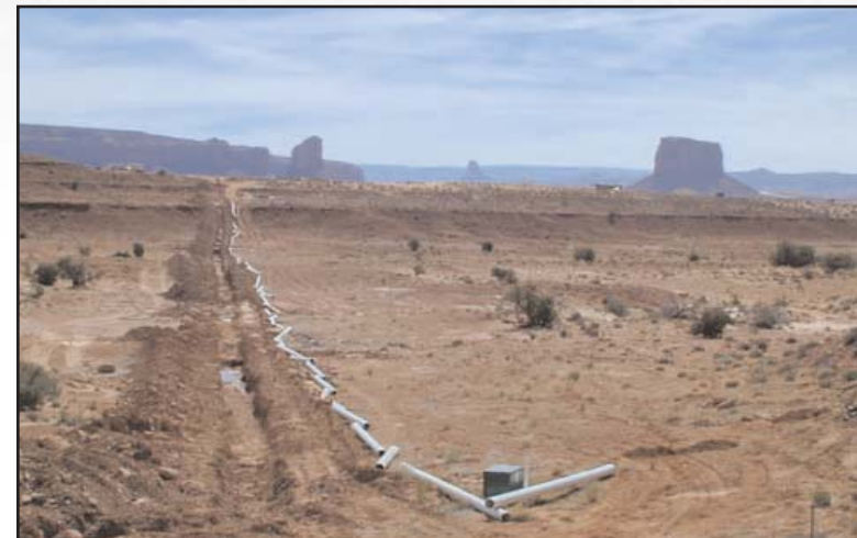
Figure 39: Waterline construction in Monument Valley, Arizona.
