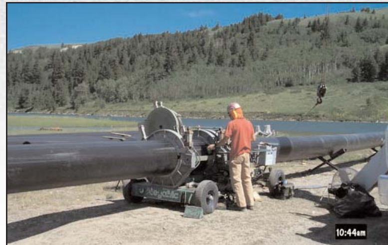
Figure 20: 22 inch HDPE pipe fused together for installation at the bottom of the lake.
