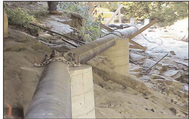
Figure 29: Pipe on piers under Straight Fork Bridge.
