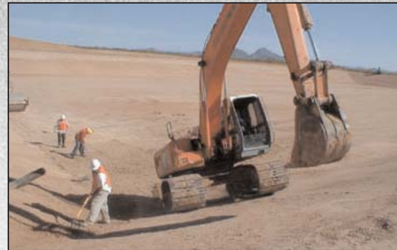
Figure 10: Preparing lagoon floor for liner expansion.
