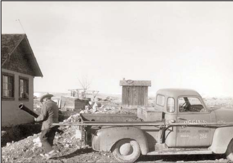
Figure 1: Construction of a septic system, 1960's
