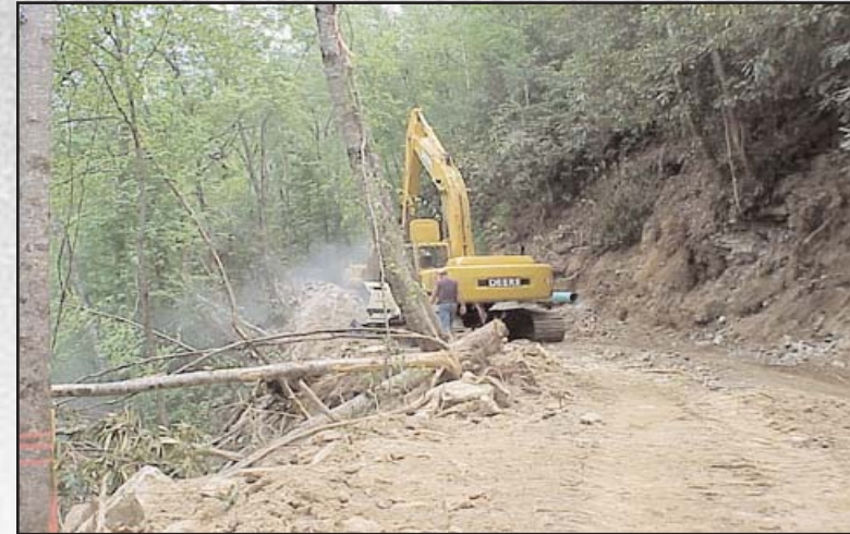
Figure 26: Mountainside installation, clearing the right-of-way.
