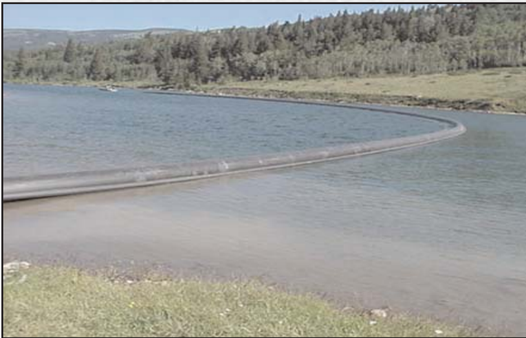
Figure 19: 22 inch HDPE pipe and 4 inch air line floating on the lake waiting to be pulled through the bore hole in the deep spot of the lake.
