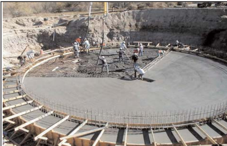
Figure 40: Concrete pour for a clarifier base on the Shiprock wastewater treatment plant.
