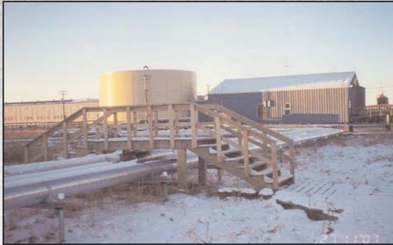
Figure 42: Vacuum sewer lines leading to a water treatment /vacuum sewer/washeteria building in Selawik, Alaska.
