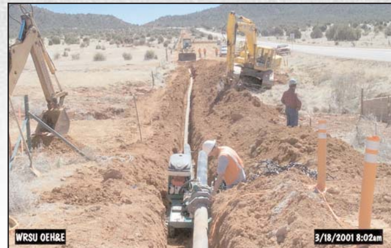
Figure 14: Over 12 miles of water transmission line was installed from Canyon Day to Cedar Creek.
