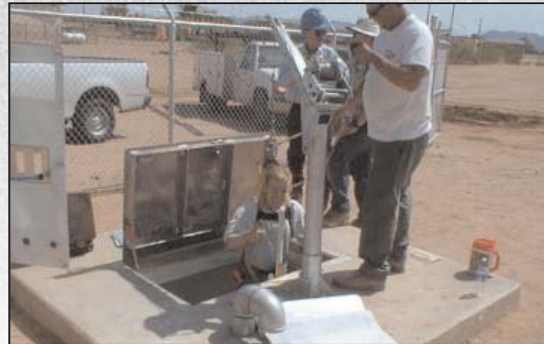
Figure 11: Project engineer Steve McGovern inspects 20 feet deep sewage lift station wet well.
