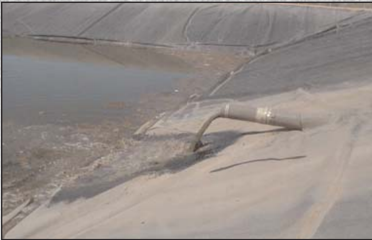
Figure 47: Wastewater flow into completed lagoon, Arizona.
