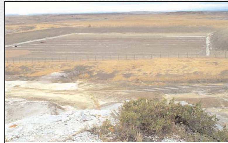
Figure 31: Completed 10-acre landfill cell with leachate collection system
