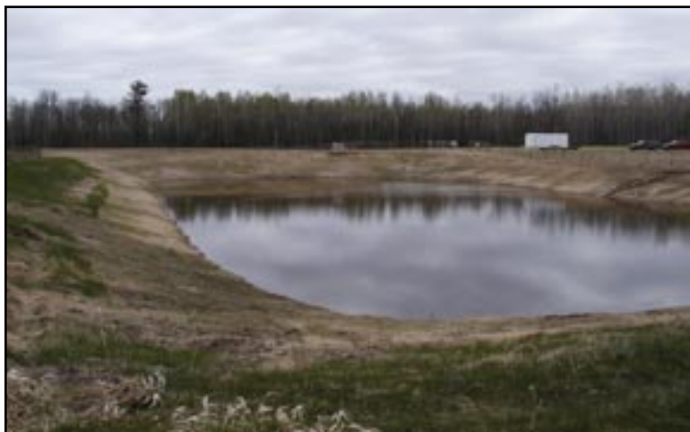
Figure 15: Renovated secondary cell in existing lagoon in East Lake, Minnesota.
