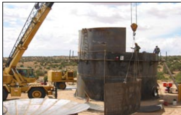
Figure 41: Construction of a 88,000 gallon water tank in White Mesa, Arizona.
