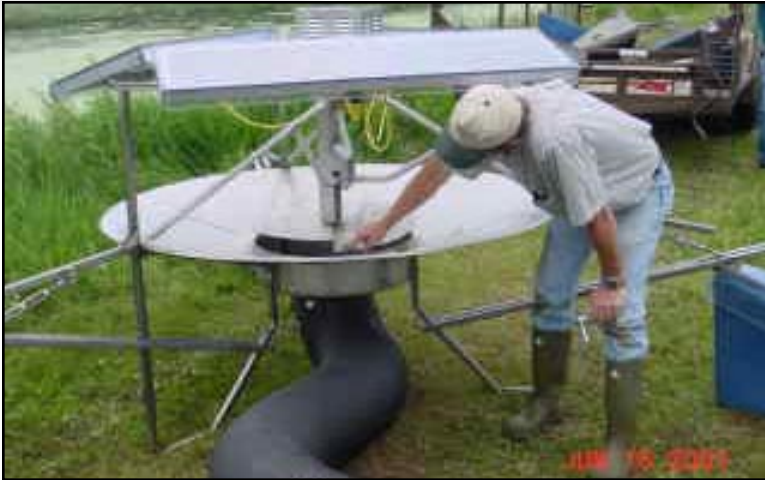
Figure 24: Pond Doctor unit being inspected by contractor.
