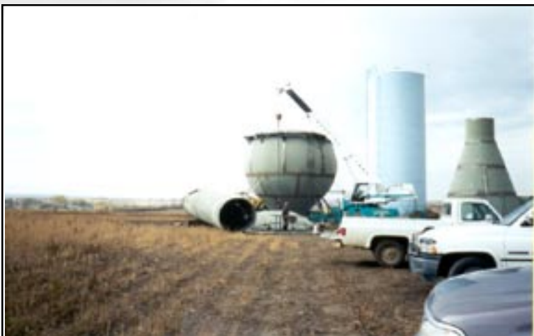
Figure 19: Erecting the middle section of the sphere.
