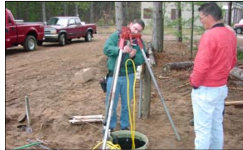
Figure 23: James Valliere, LDF Assistant Operator, and contractor setting up hoist to remove the grinder pump, Lac du Flambeau, MI.
