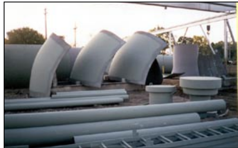
Figure 18: Water sphere components ready to be erected and welded.
