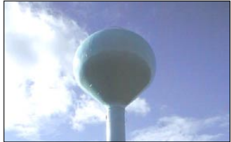
Figure 34: Completed 250,000 gallon elevated water tower.
