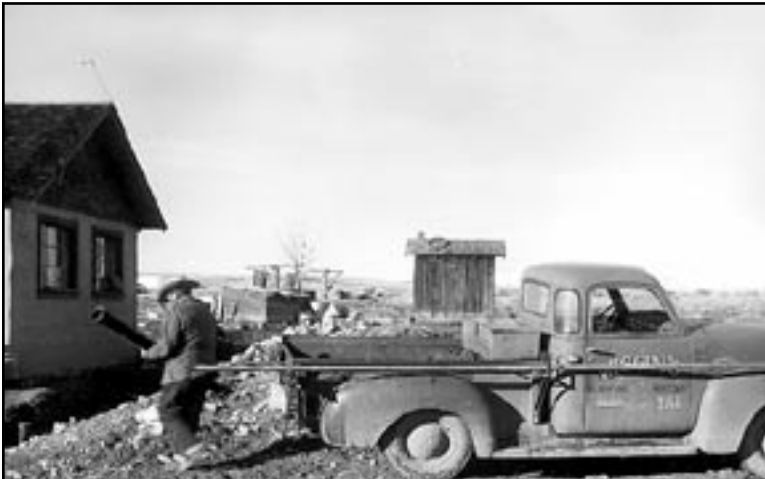
Figure 1: Construction of a septic system, 1960's
