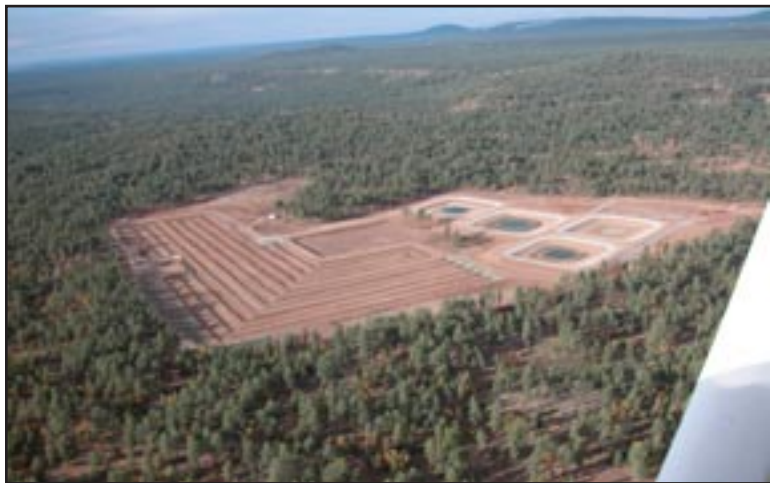
Figure 35: Aerial photo of the recently constructed wastewater treatment facility at Hon Dah, Ft. Apache Indian Reservation, Arizona.
