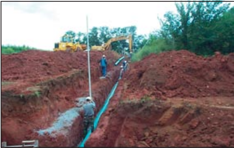
Figure 33: Checking sewer main grade to accurately tie into existing sewer by old lagoon.
