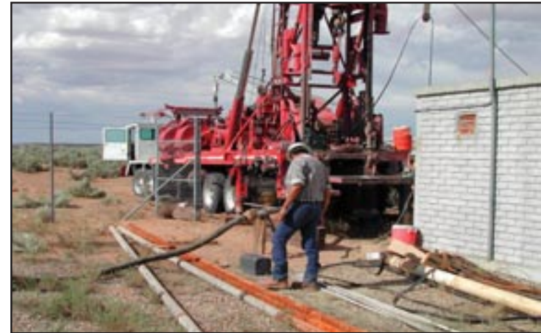
Figure 46: Chester Lapahie of the Farmington, New Mexico field office does test pumping at Ojo Encino on the Navajo Reservation, New Mexico.
