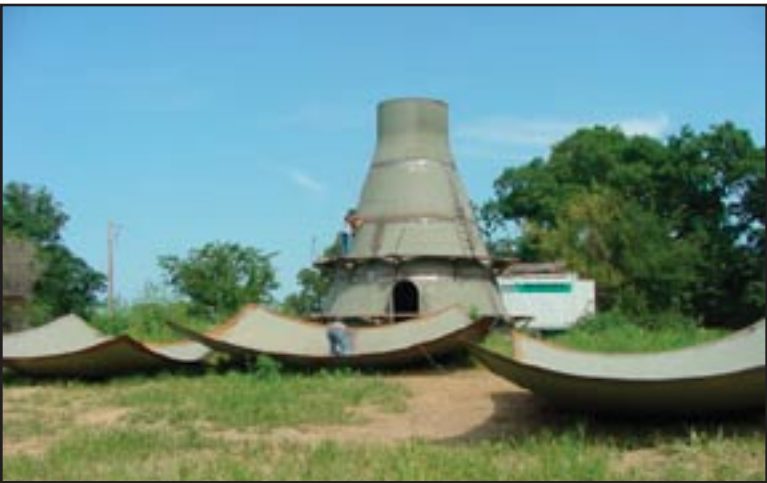
Figure 42: 300,000 gallon water sphere being assembled at the Sac and Fox settlement, Iowa.
