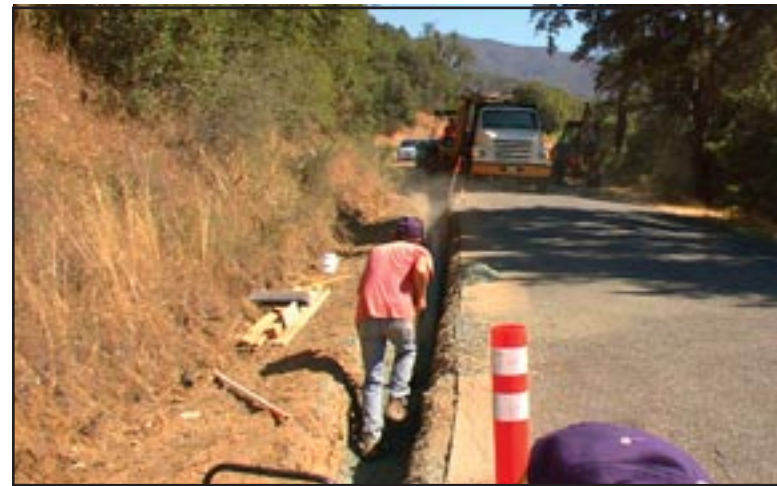
Figure 18: 8-inch PVC pipe installation with pipe embedment.
