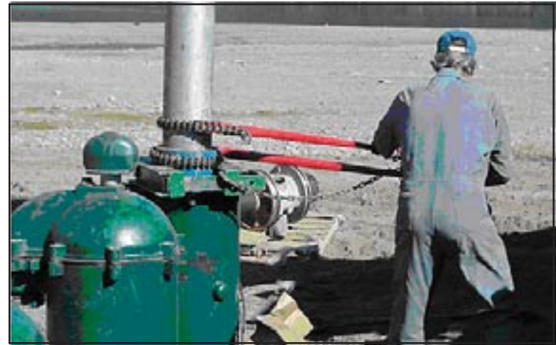
Figure 10: Intake pump fittings and pipe being assembled which the connections torqued to 3,500 ft-lb.
