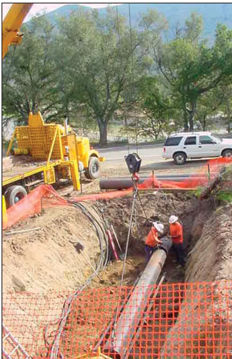
Figure 7: : Road bore as part of a 4 mile water main installation on the La Jolla Reservation, California.
