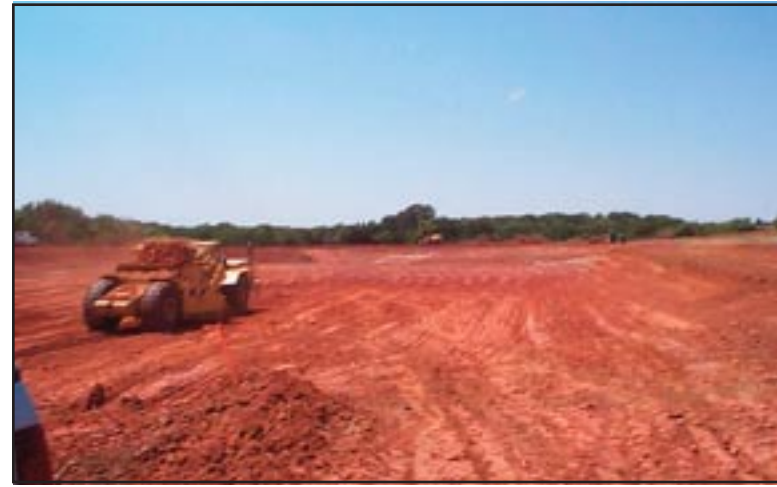
Figure 30: Initial excavation and berm compaction of lagoon.
