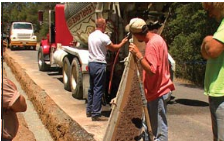
Figure 19: Cement slurry mix poured over pipe embedment along Dewell extension.
