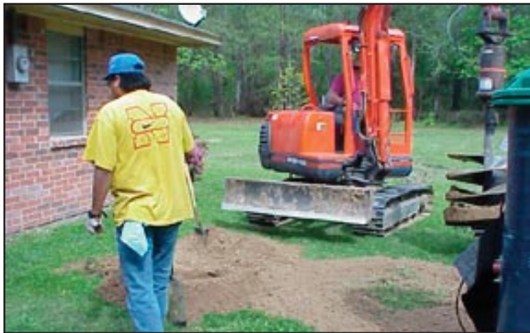
Figure 24: Tribal crew installing individual grinder lift station.
