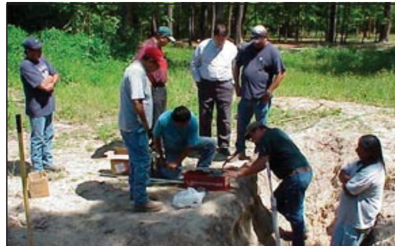
Figure 25: Tribal crew pressure testing the small diameter pressure sewer main.
