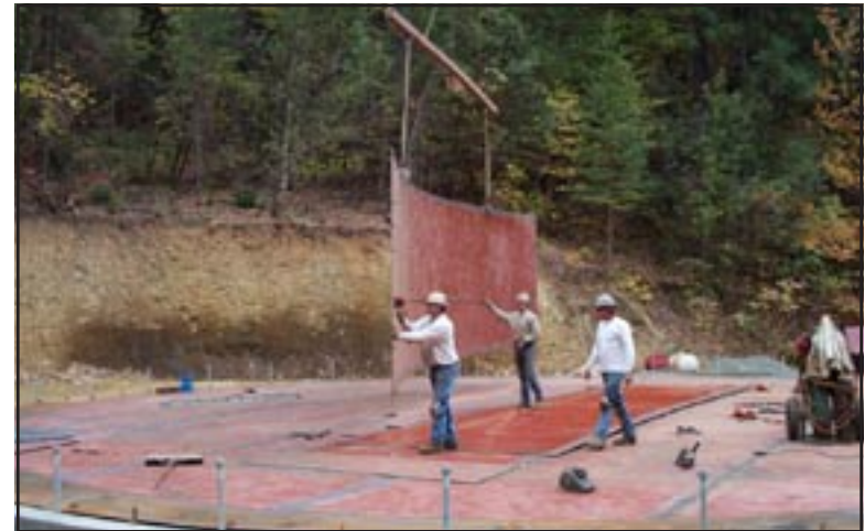
Figure 14: 1 million gallon water storage tank under construction.
