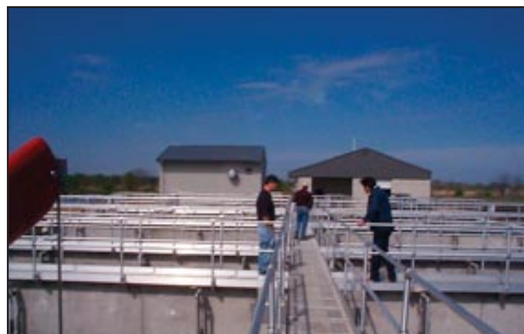
Figure 8: Startup of the mechanical wastewater treatment plant at Sac and Fox, Iowa.
