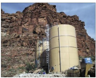
Figure 16: New 108,000-gallon water storage reservoir.
