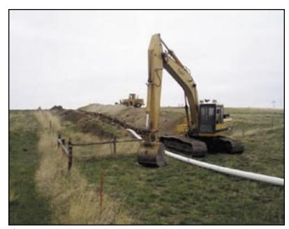
Figure 11: Waterline installation.
