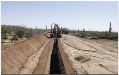
Figure 23: Laying HDPE pipe.
