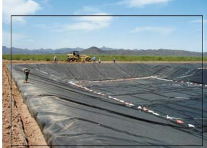
Figure 19: Anchor trench installation.
