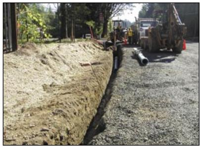
Figure 29: 8" PVC water main installation.
