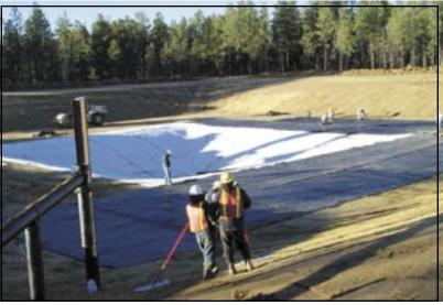
Figure 12: Installation of geosynthetic clay liner in a fermentation pond.
