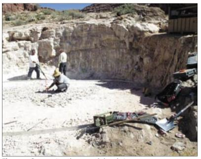
Figure 17: Construction of a new tank foundation.
