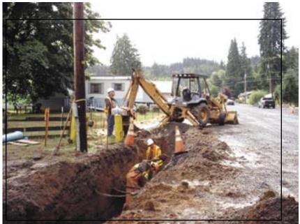
Figure 28: 8" PVC water main installation.
