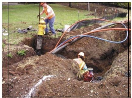
Figure 26: Hydrant installation.
