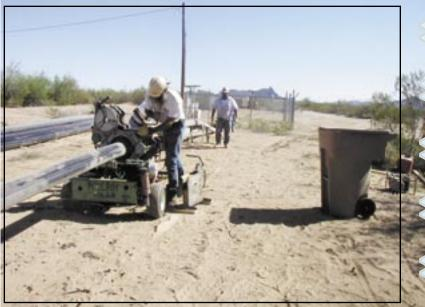
Figure 22: Fusing HDPE pipe.
