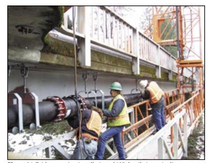
**Figure 34:** Bridge crossing installation of 10" ductile iron pipeline, California.
