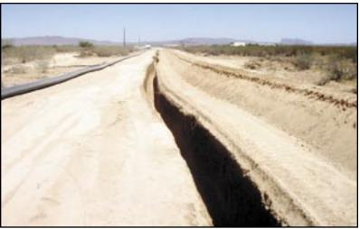
Figure 24: Sewerline trench.
