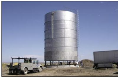
Figure 10: New 300,000-gallon stainless steel reservoir.
