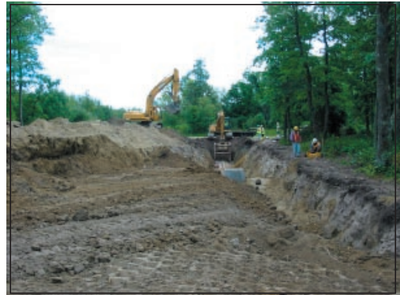
Figure 17: Leech Lake Band Public Works staff installing gravity sewer main .
