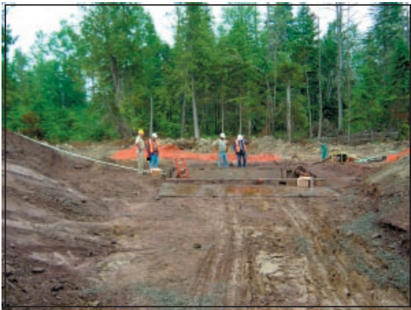
Figure 35: Excavation for wet well lift station, Pleasant Point, Maine.
