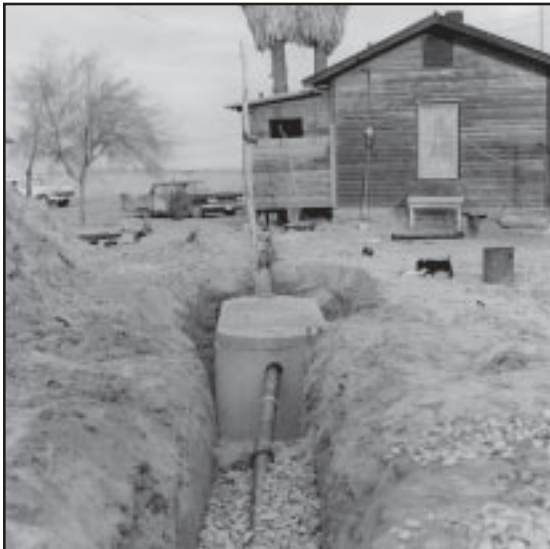
Figure 1: Construction of a septic system, 1960's.
