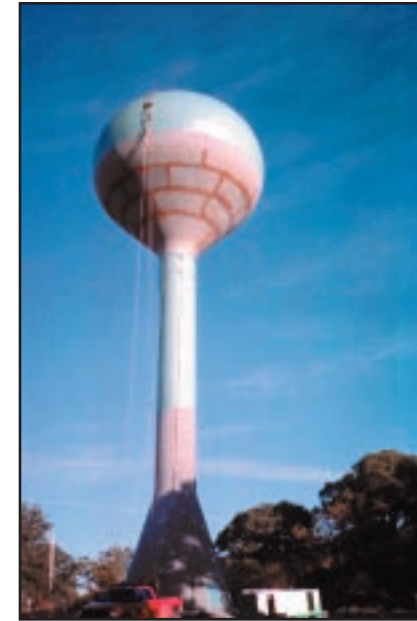
Figure 38: Almost completed water sphere for Sac and Fox, Iowa.
