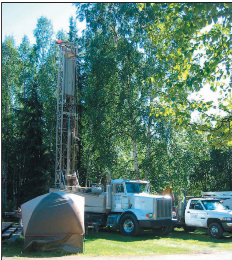
Figure 7: Water well drilling in Fairbanks, Alaska.
