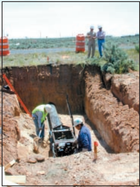
Figure 23: Preparing for a road bore to extend the 14 inch waterline.
