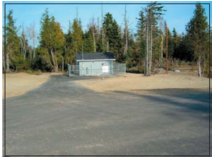
Figure 36: Completed lift station, Pleasant Point, Maine.
