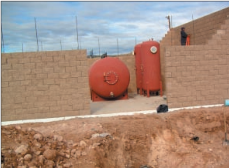
Figure 9: Jemez filtration installation during building construction.
