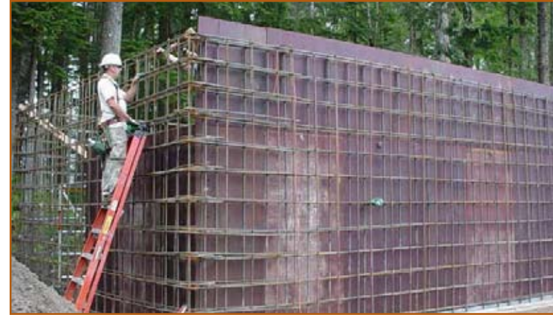
Figure 15: Sedimentation tank rebar and forms. An estimated 80,000 pounds of rebar was required for the construction of the sedimentation tank and building.
