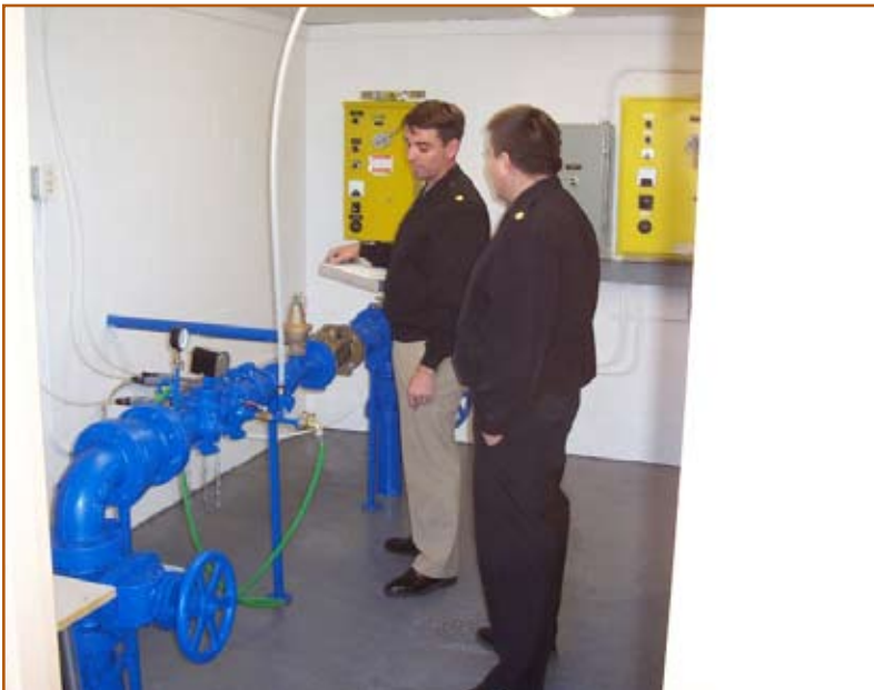
Figure 4: IHS engineers at the final inspection for pumphouse expansion for Desmet community, ID.
