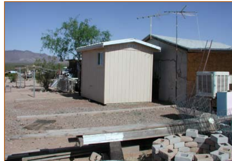
Figure 32: Finished and installed modular bathroom.
