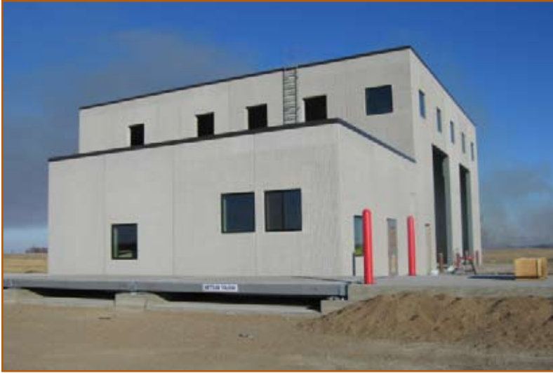
Figure 23: Transfer station near completion.
