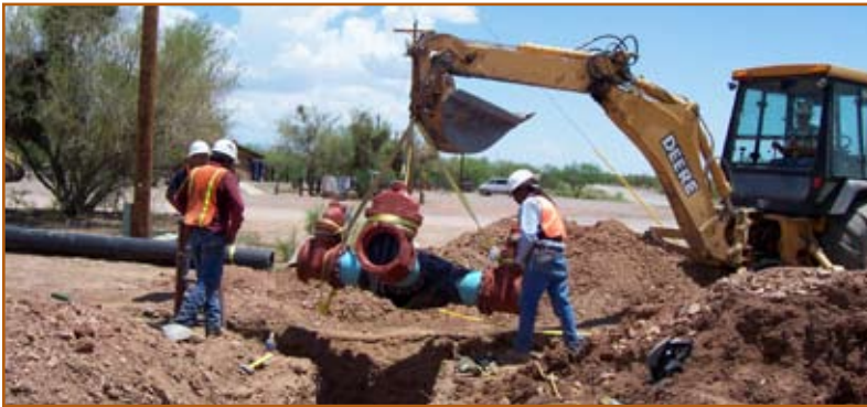
Figure 25: Installing 24-inch tee and valve assembly.
