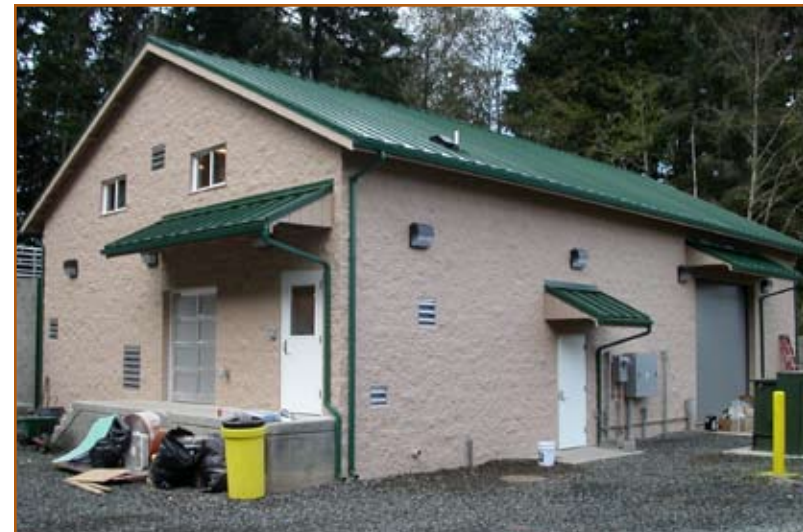
Figure 16: New Makah WTP near completion.
