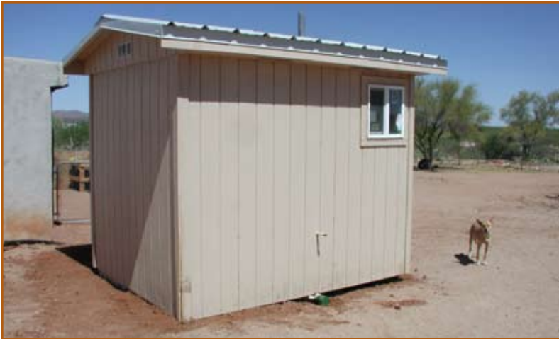
Figure 31: Back of modular bathroom.
