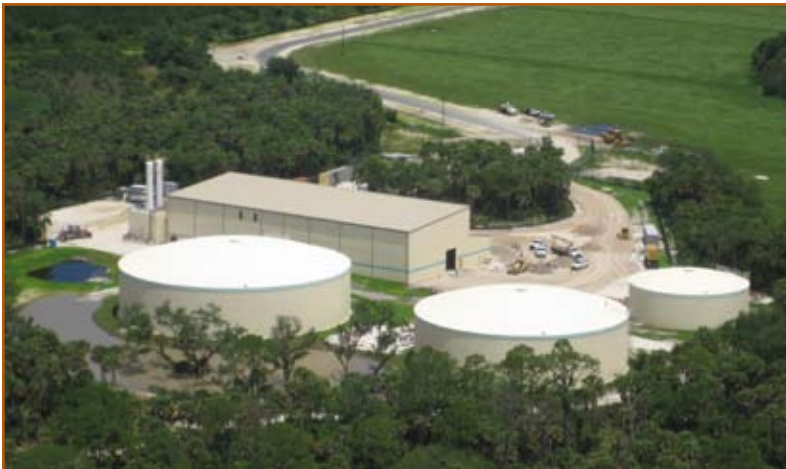
Figure 40: Aerial view of the newly constructed $30 million Brighton WTP owned and operated by the Seminole Tribe of Florida.
