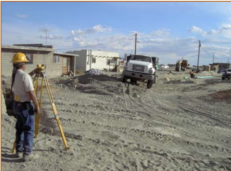
Figure 9: Engineering technician Erwin Tewa shoots grade on the new 8" PVC sewer line extension in Shungopavi Village.
