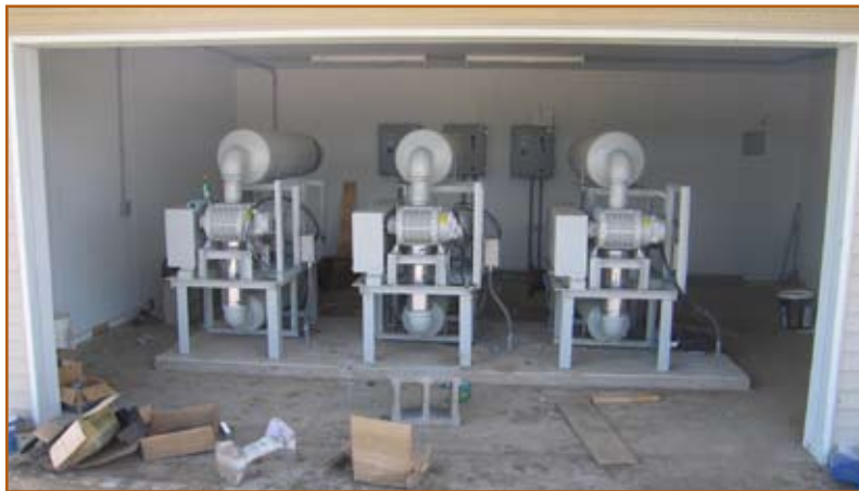
Figure 19: 18-foot x 24-foot blower building under construction.
