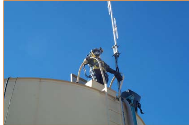
Figure 3: Tank diver inspecting and cleaning water storage tank, NM.
