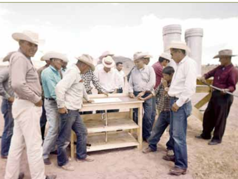
Homeowner Training, 1960's.
