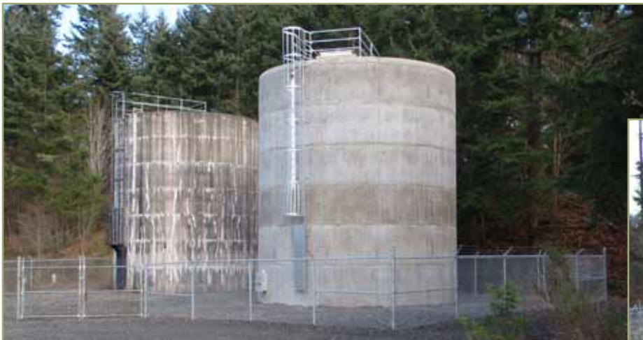
Completed and existing water storage tank.
