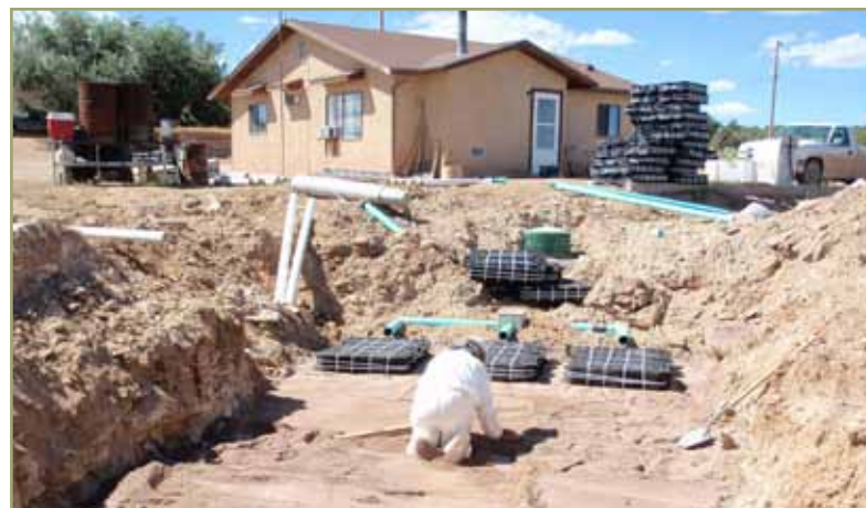
Septic tank and drainfield installation, Chinle, Arizona.
