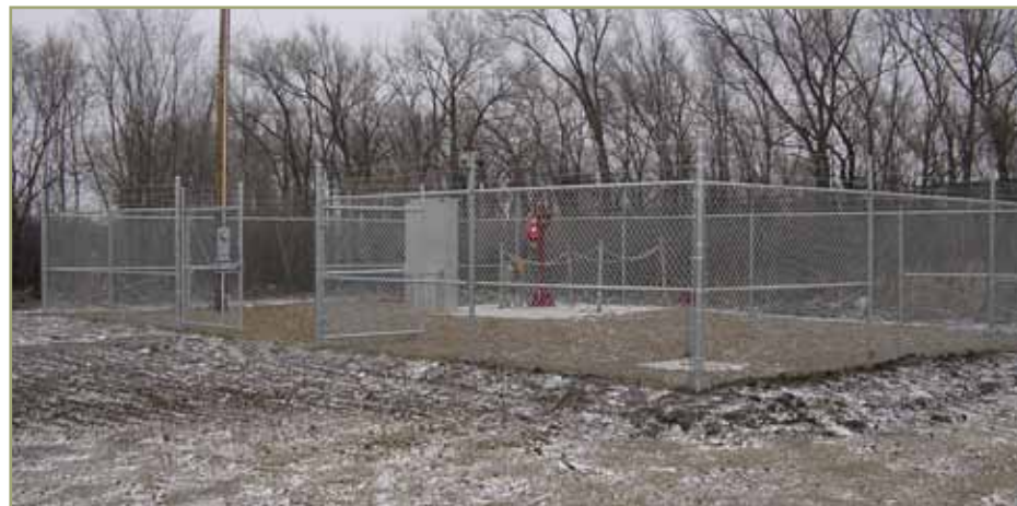
Exterior of the renovated lift station building.
