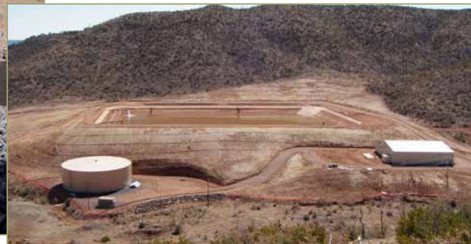
Overall of the completed water treatment plant.
