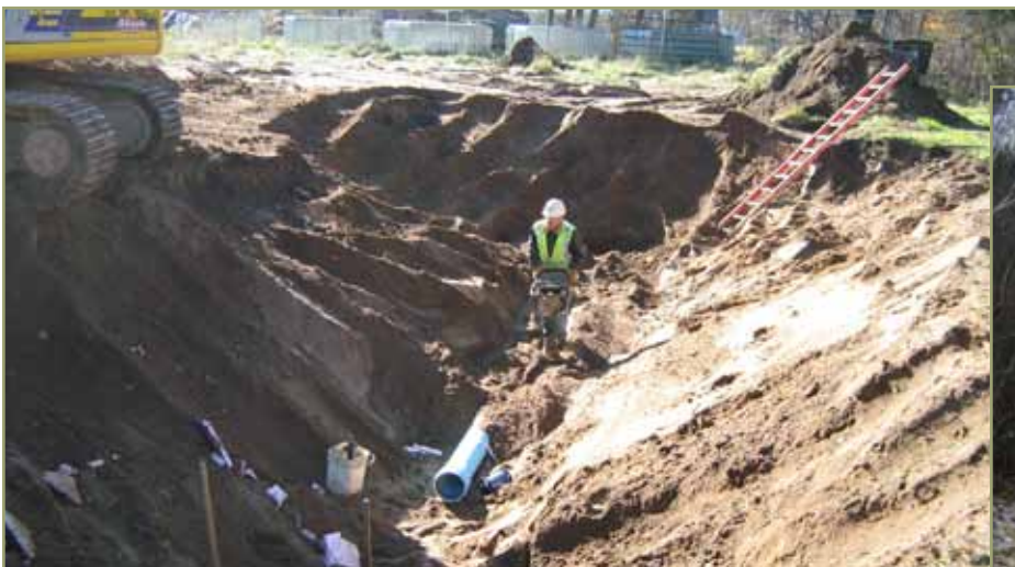
Soil compaction in the waterline trench.
