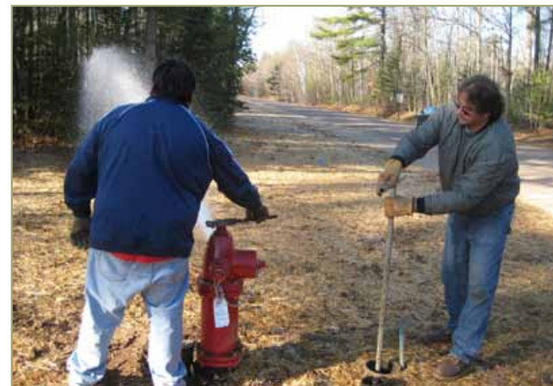
Testing the fire hydrant.
