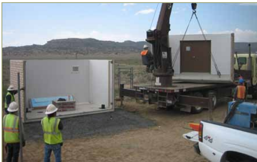
Precast booster pump station, Burnt Corn, Arizona.
