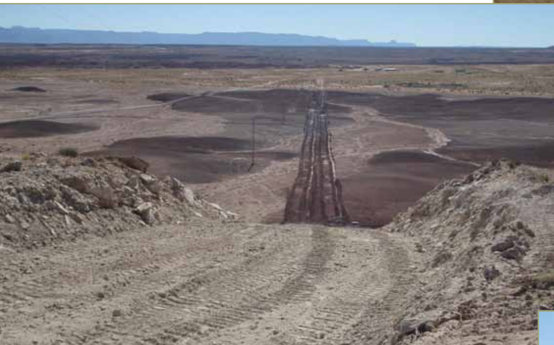
Clearing of the right of way for the waterline project.
