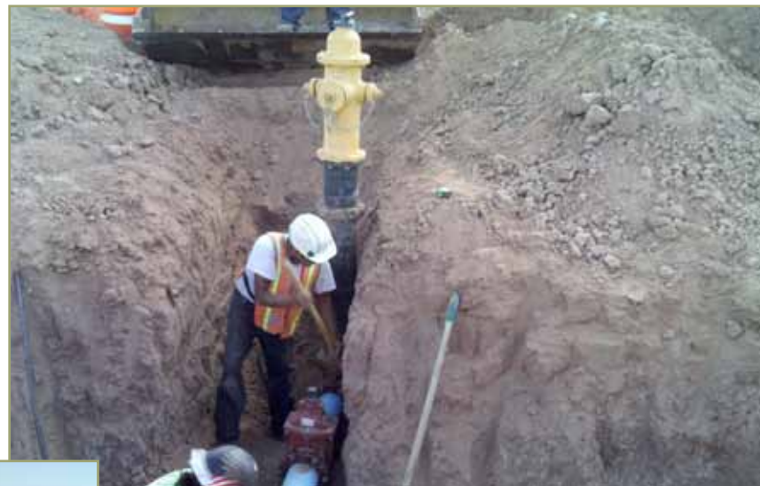
Construction of the water distribution line.
