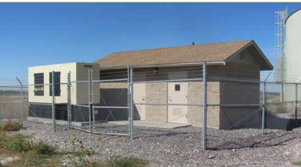
Cemetery Road pump house on the Fort Hall Indian Reservation, Idaho.
