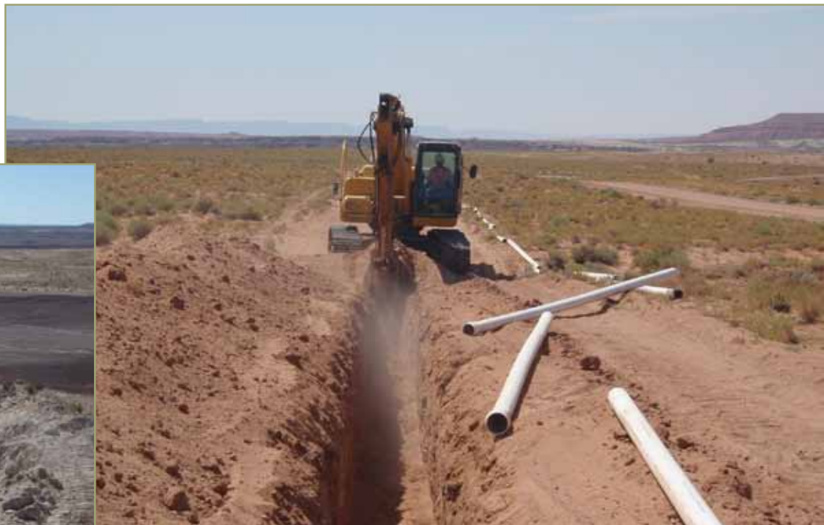
Construction of the waterline trench.
