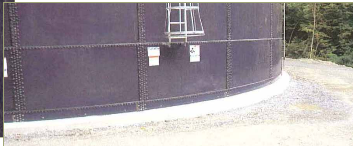
The reconstructed tank and foundation.
