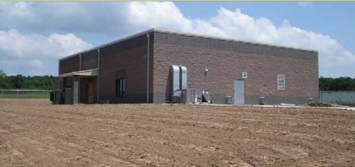
Completed water treatment plant.
