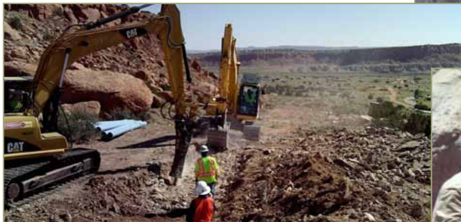
Clearing the right of way and rock excavation for the tank.
