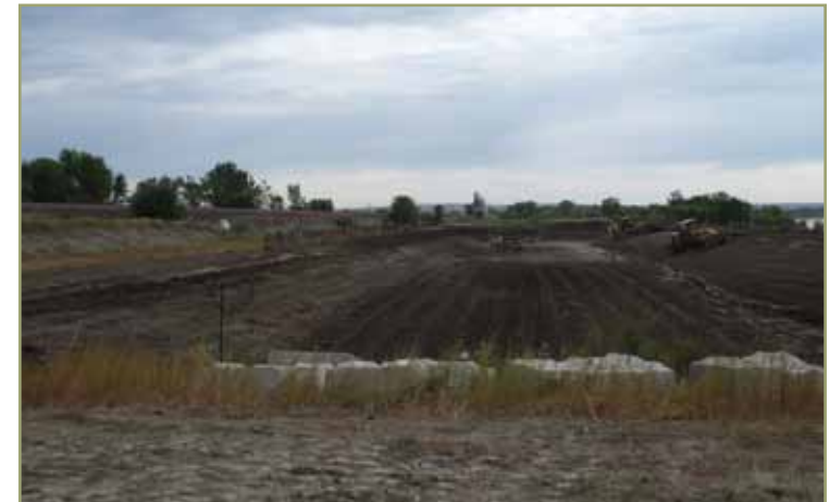
Reconstruction of the embankment.
