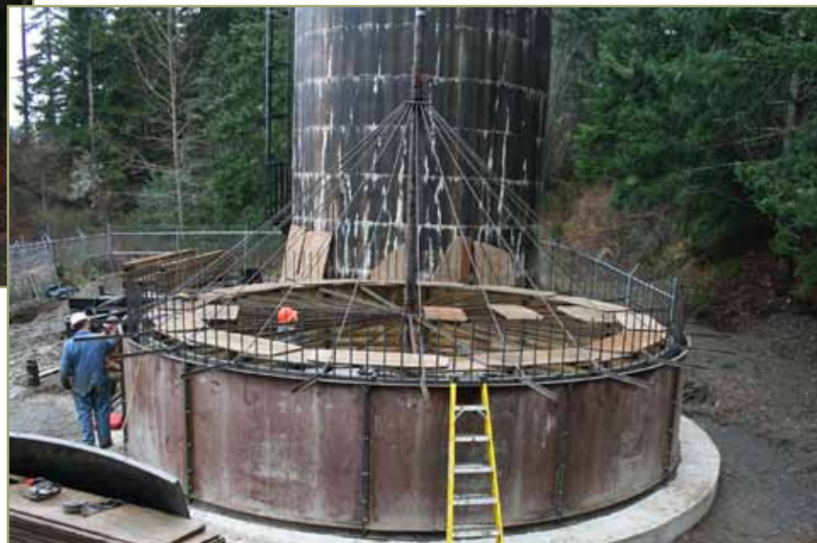
Construction of the concrete tank.
