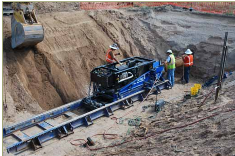
24" Road bore under I-25 for the Sandia Pueblo, New Mexico.
