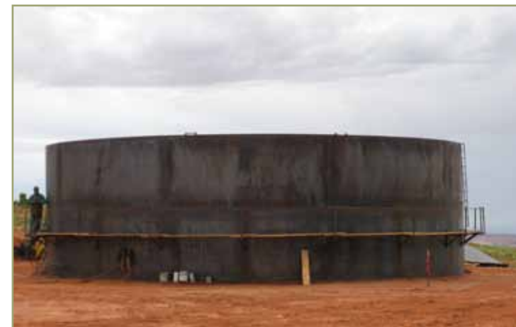
500k water tank construction, Sweetwater, Arizona.
