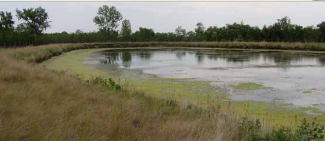
The lagoon before the repair
