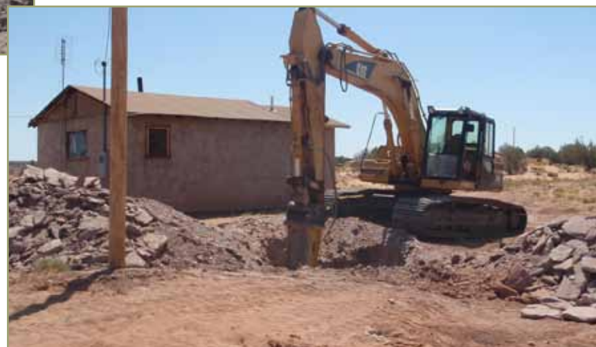
Installation of a septic tank drainfield system. 1
