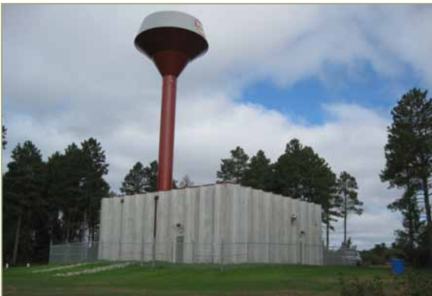
Community water system for the Leech Lake Band of Ojibwe, Minnesota.
