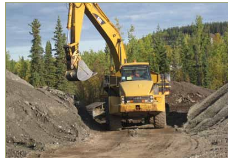
Removal of soil to complete the lagoon.
