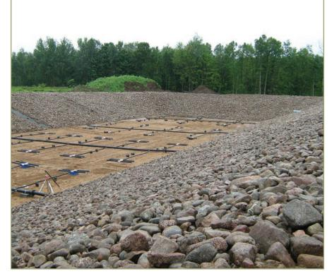
Installation of diffusers in the new aerated lagoon cell, Wisconsin.
