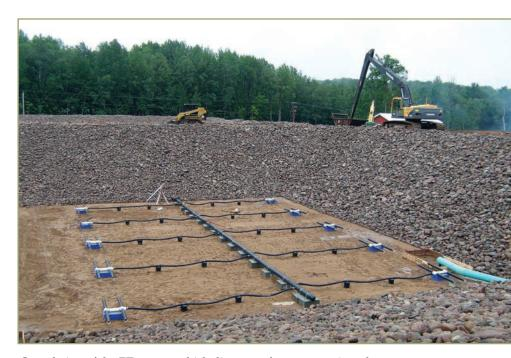
Completion of the ET system which disposes of wastewater into the atmosphere through evaporation.
