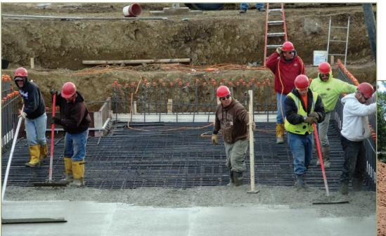
Contractor pouring the foundation for a 100k gallon buried concrete reservoir for on the Lake Traverse reservation, South Dakota.
