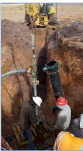
Installing pitless adapter on well casing, Utah.
