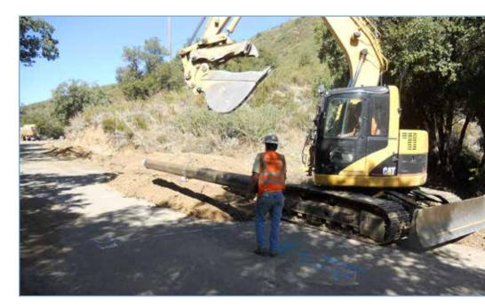
Water pipe in steel casing being installed at culvert crossing.
